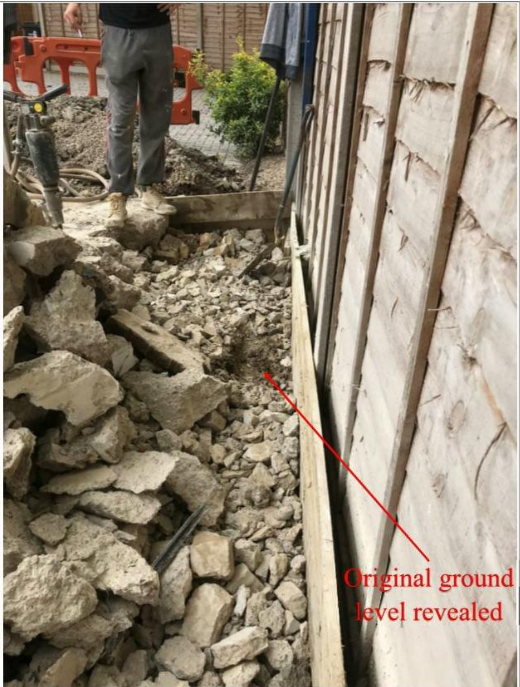
Photo 5: Removal of concrete base slab and arisings close to boundary fence to reveal original ground level
