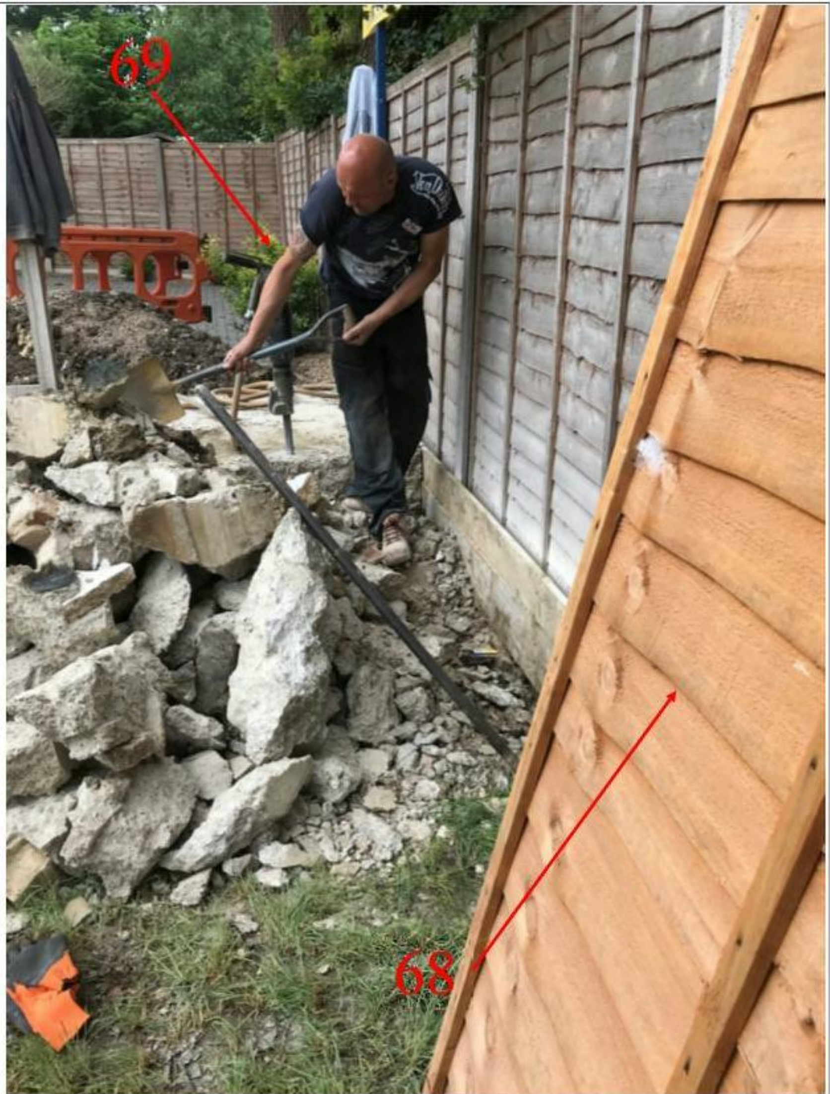
Photo 4: Arisings from the breaking up of the concrete base slab being removed by hand close to boundary fence and trees to investigate potential direct root damage
