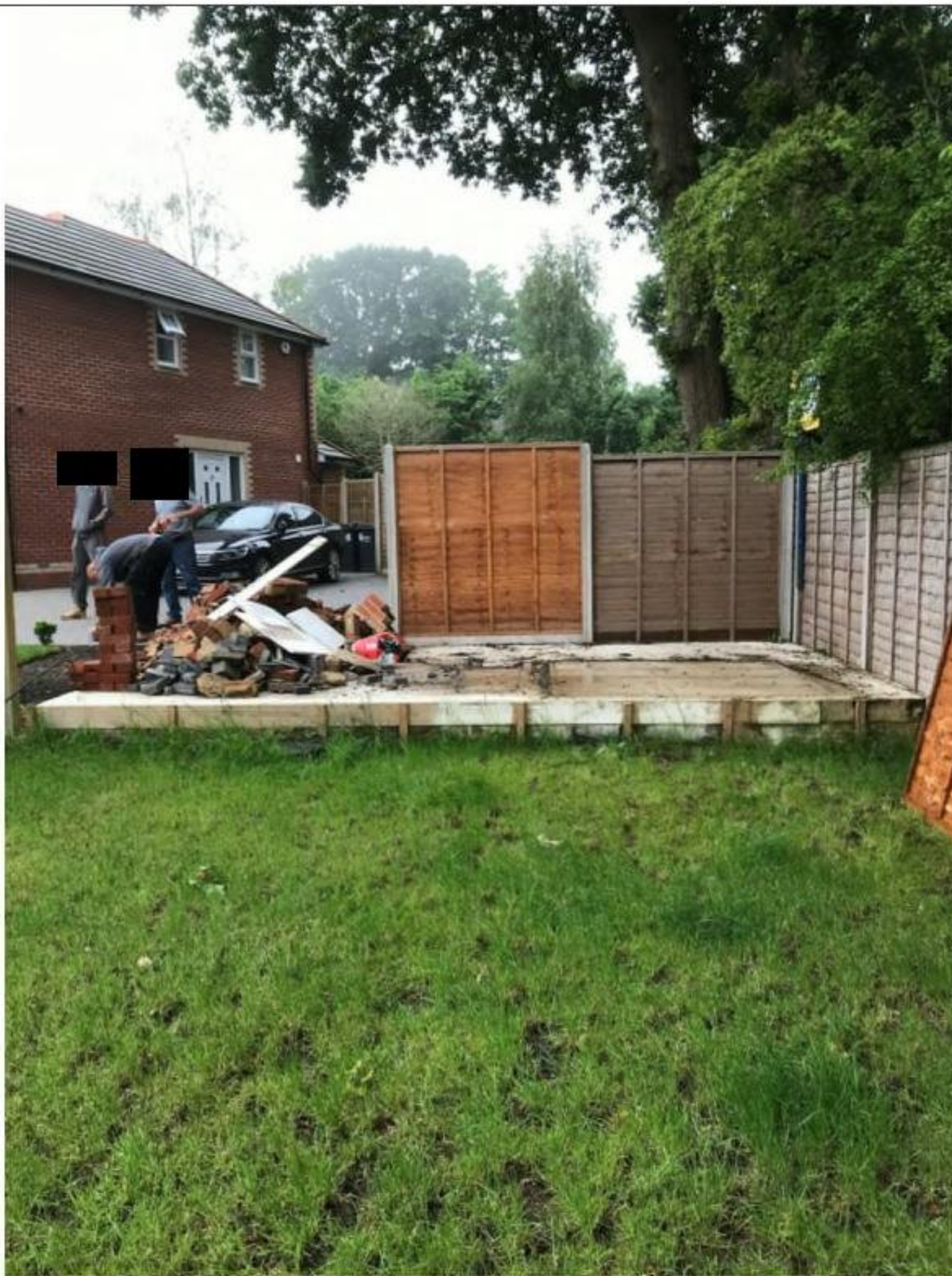
Photo 1: Concrete slab base prior to the start of removal works
