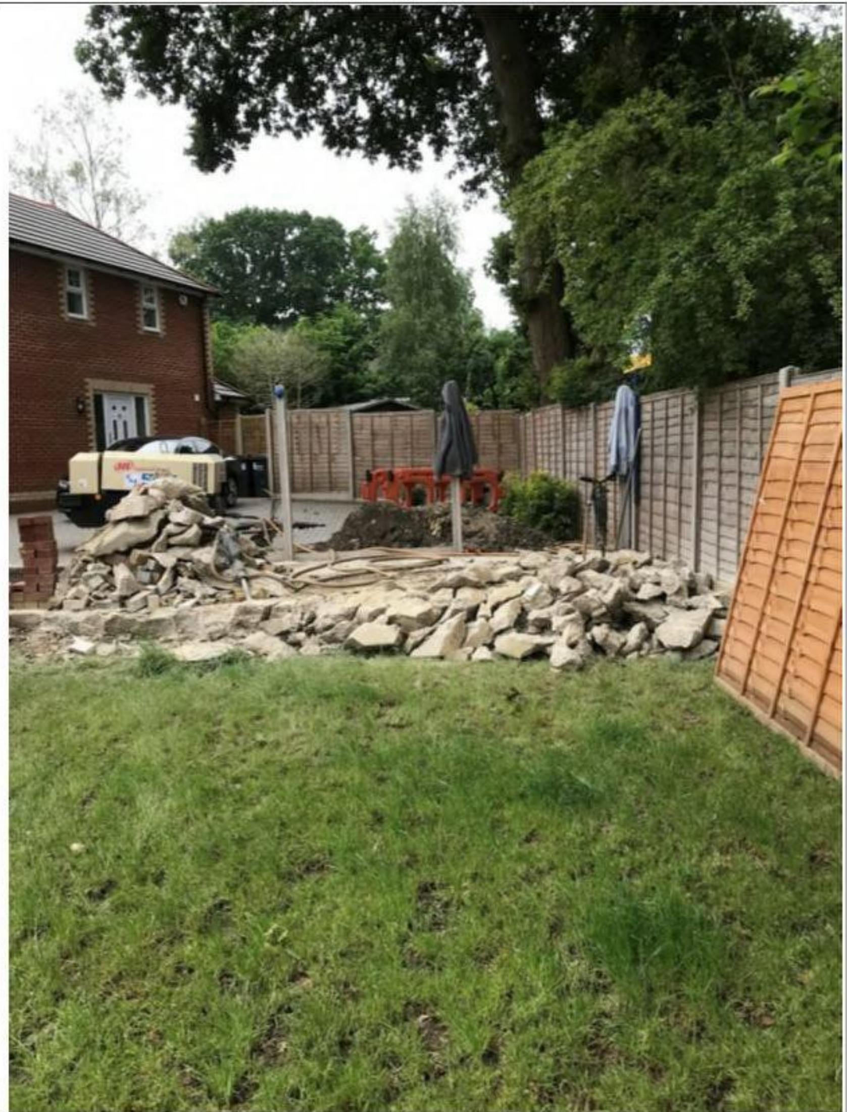
Photo 3: Concrete slab base partly broken up, with arisings beginning to be stacked on remaining part of slab
