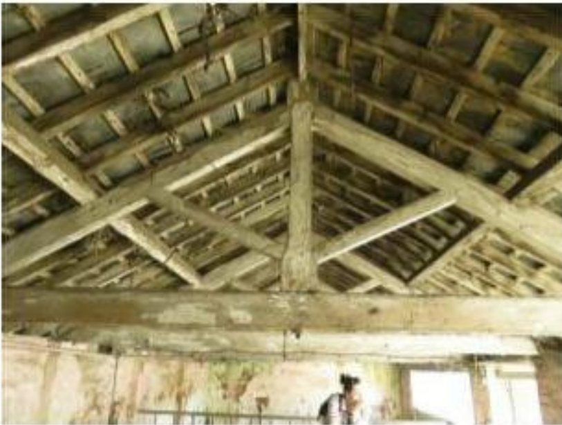
View of Timber Roof Truss
