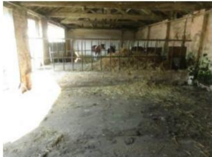
Internal view looking West
