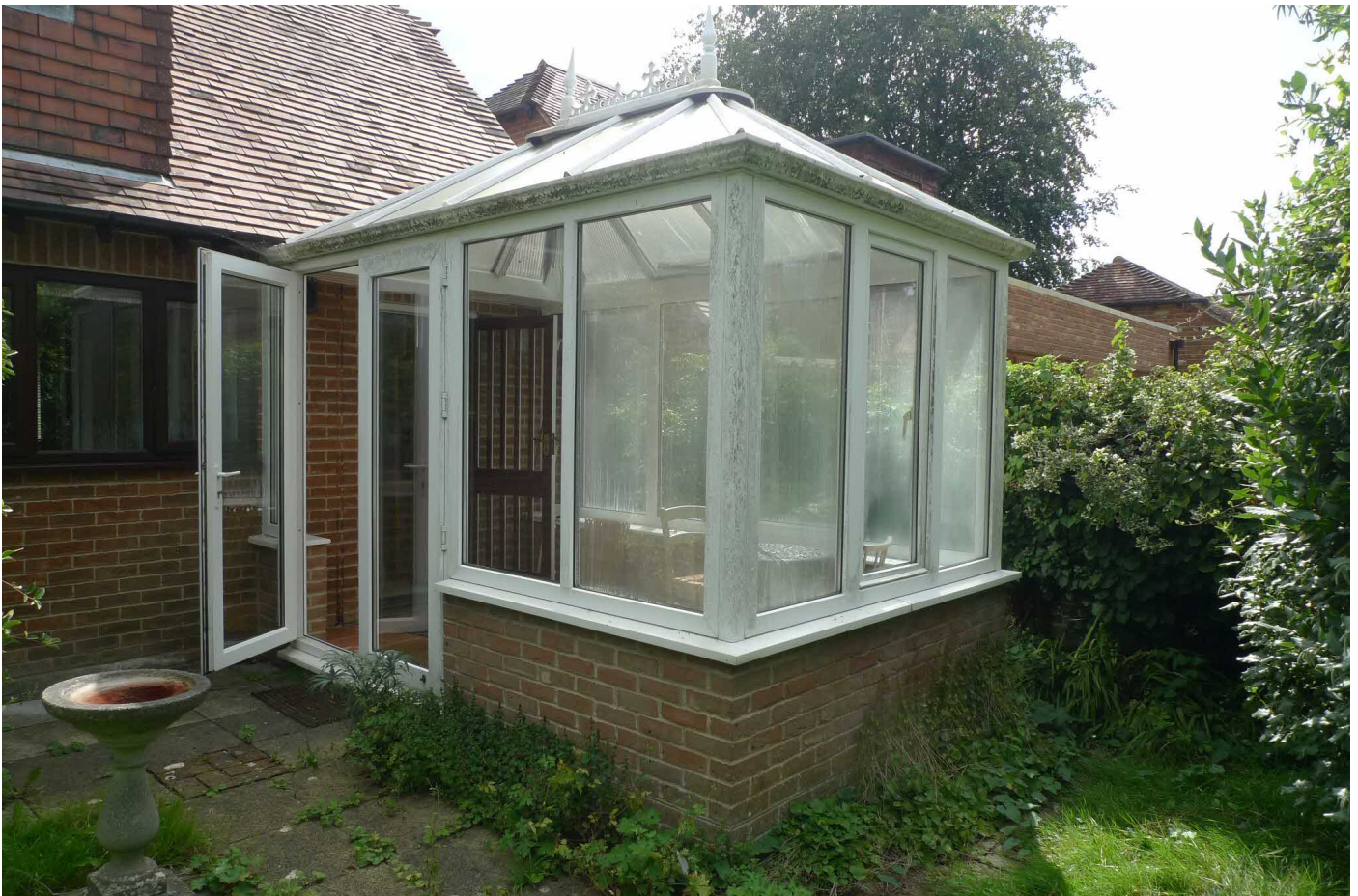
The existing rear conservatory
