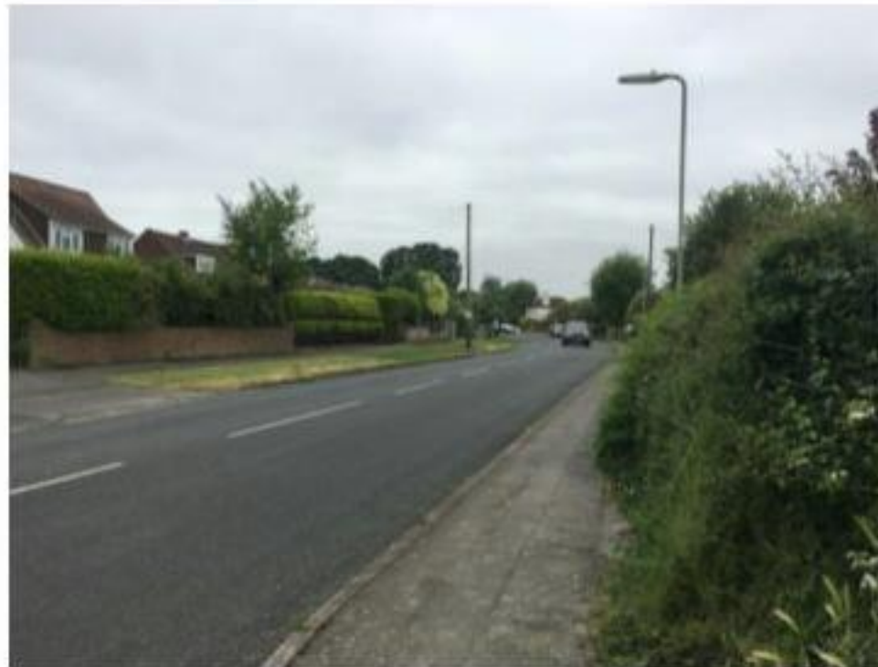
Photograph 1: Sinah Lane Conditions
