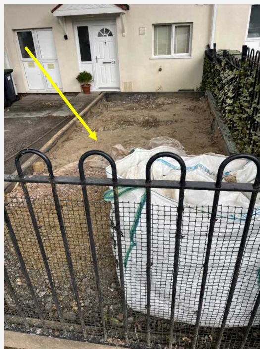
T1 Looking to the East to loose raised driveway
