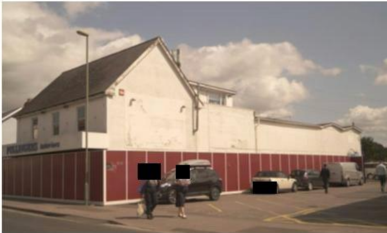
3.4.1| No. 108 Elm Grove - existing retail unit facing street
