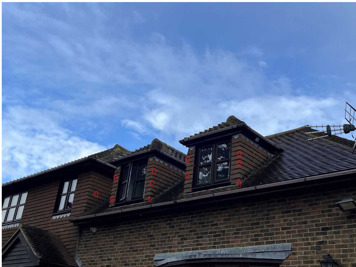
Figure 7. Southern elevations looking northwest: Red arrows indicate potential openings into under-tiles spaces.
