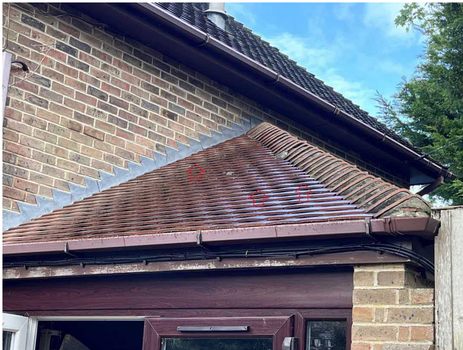
Figure 9. Converted garage looking northwest: Red arrows indicate potential openings into under-tiles spaces.
