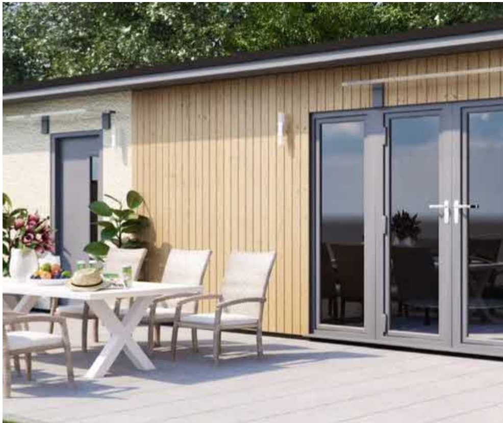
Diagram 3: example photograph showing the mix of proposed materials, grey anthracite windows and doors, render and vertical timber cladding.
