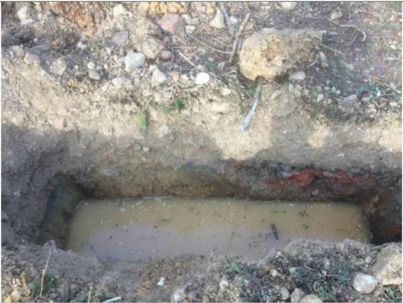
PLATE 3 – TP1 at start of soakaway test
