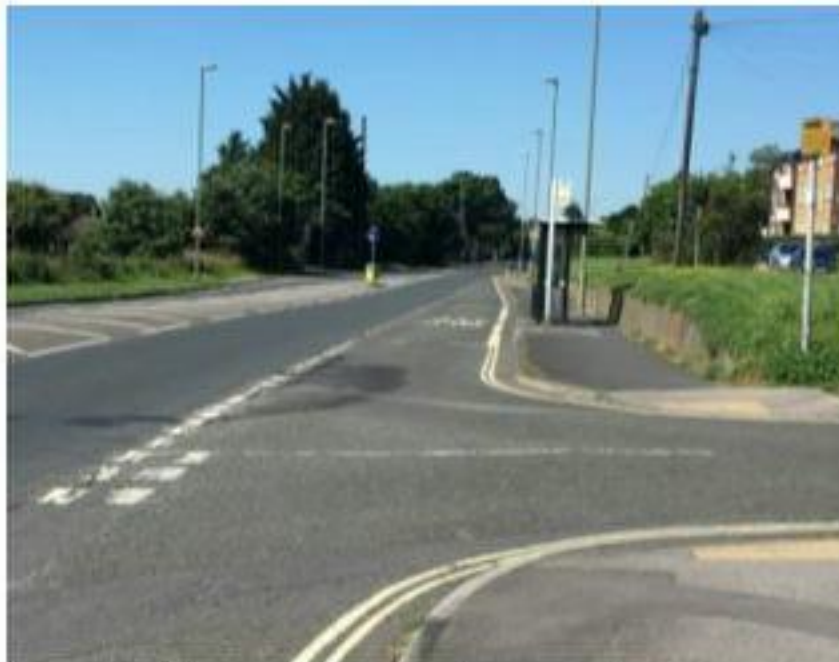
Photograph 8: Rectory Avenue NE-bound
