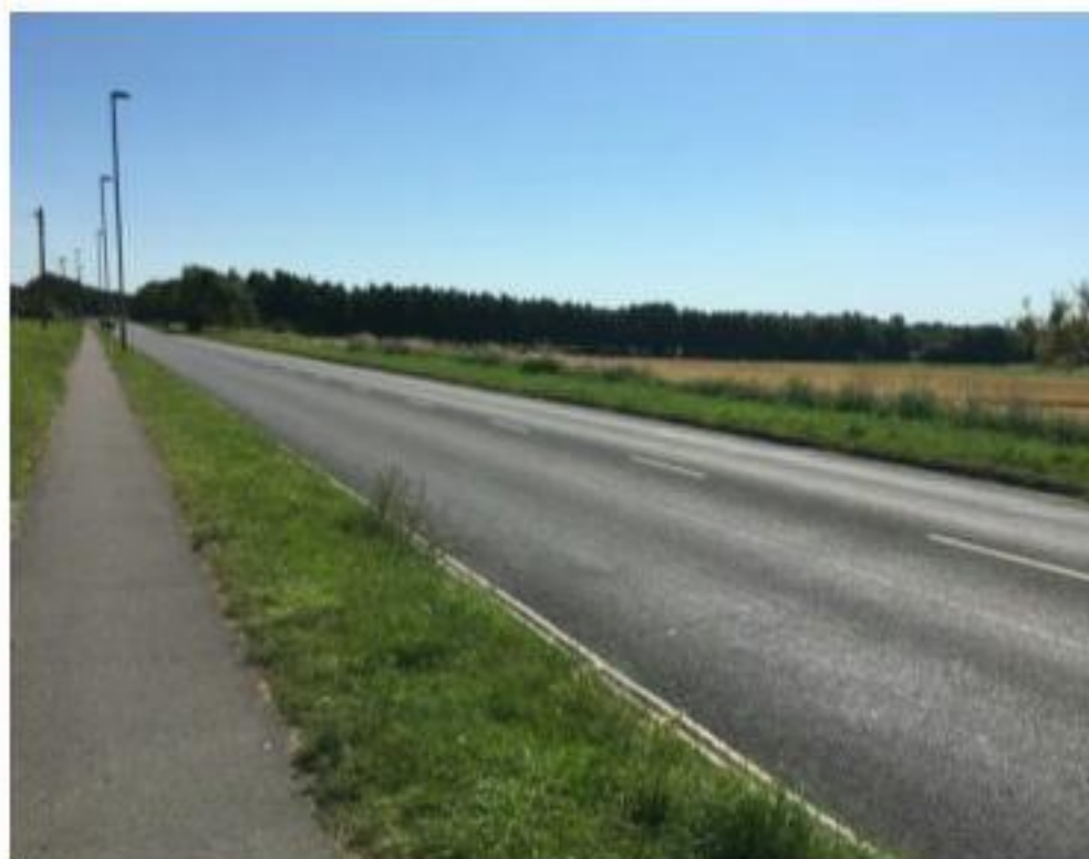
Photograph 10: Havant Road (A2030) Environment
