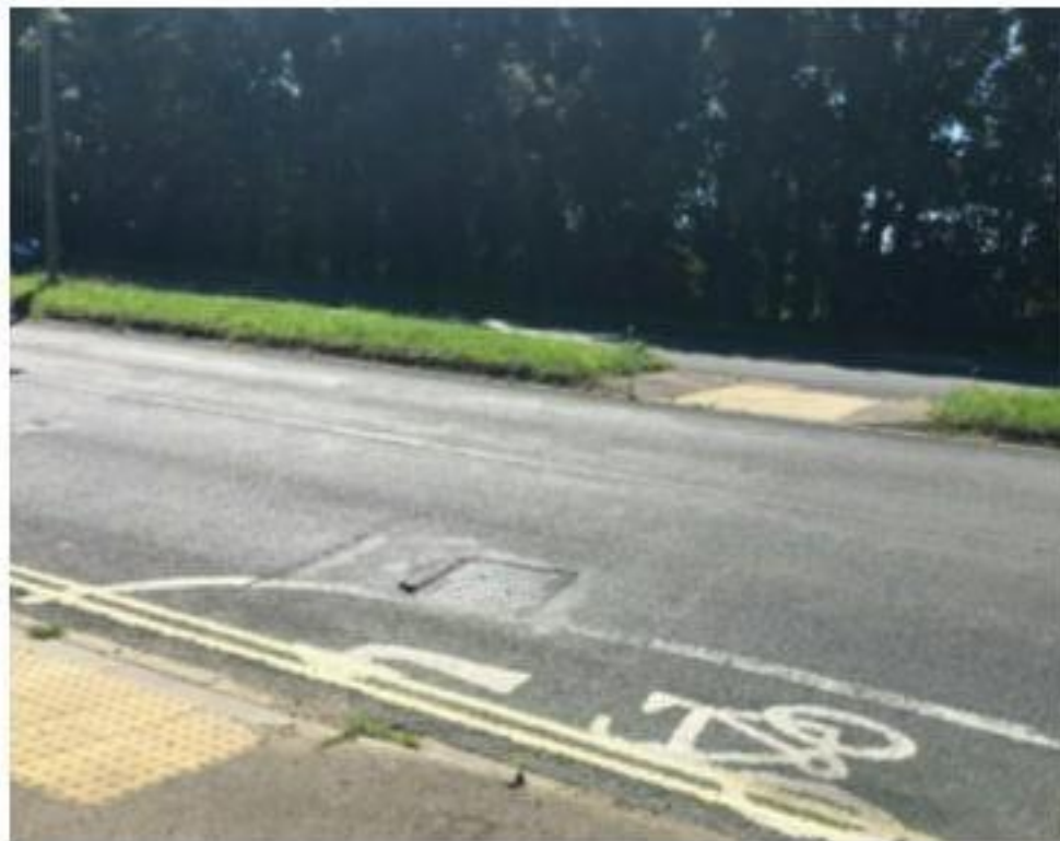
Photograph 3: Existing Pedestrian Crossing facilities
