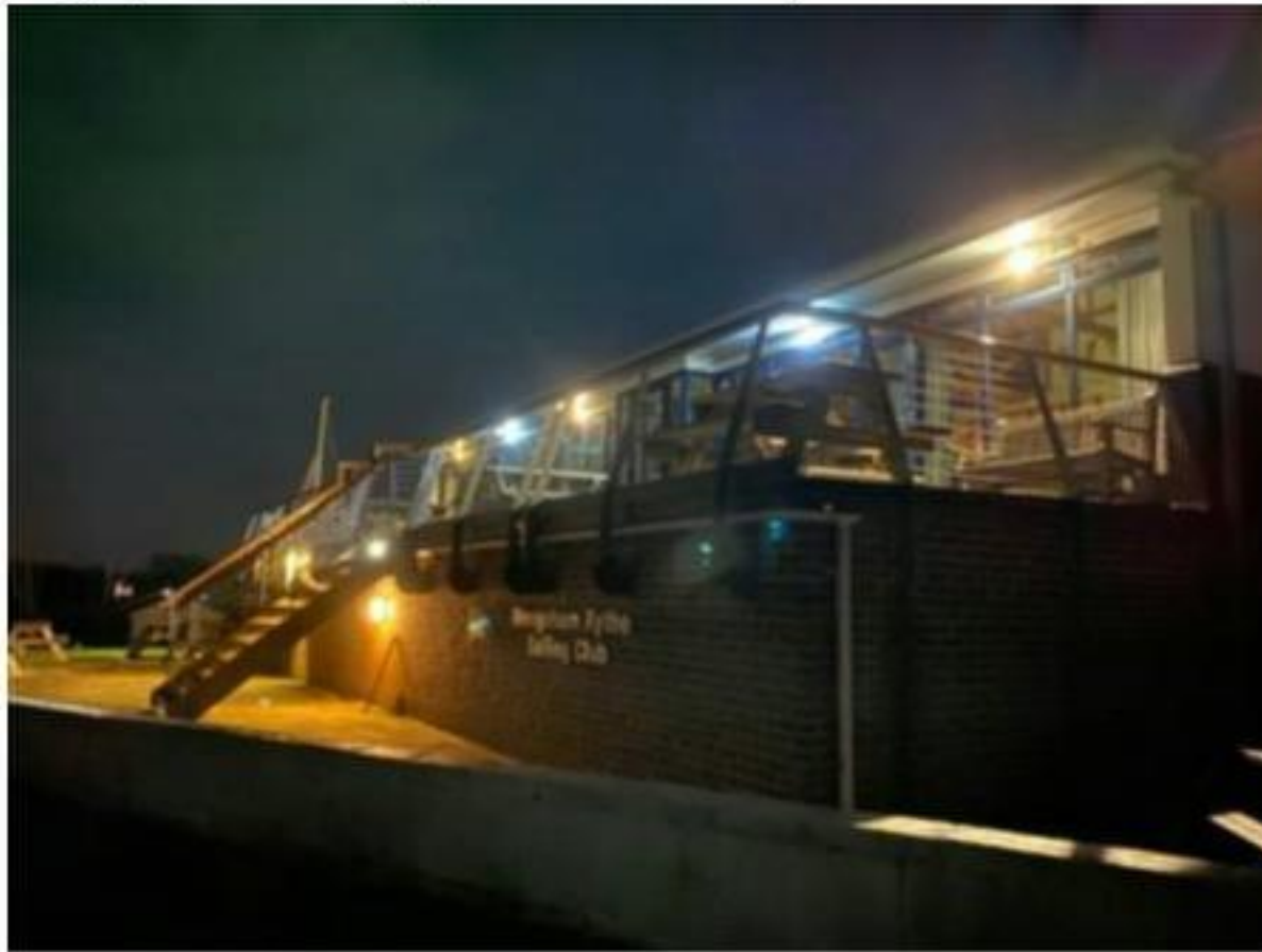
Photo 10. Security lights at Mengham Rythe Sailing Club facing directly out across the harbour and the mouth of My Lord's Pond opposite the Tournerbury Woods Estate.
