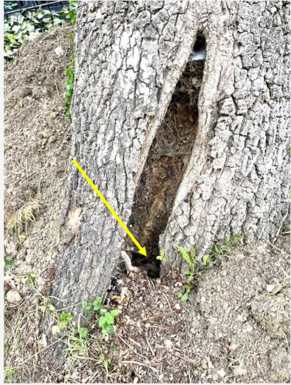
T1 Extensive basal cavity to Northwest side.
