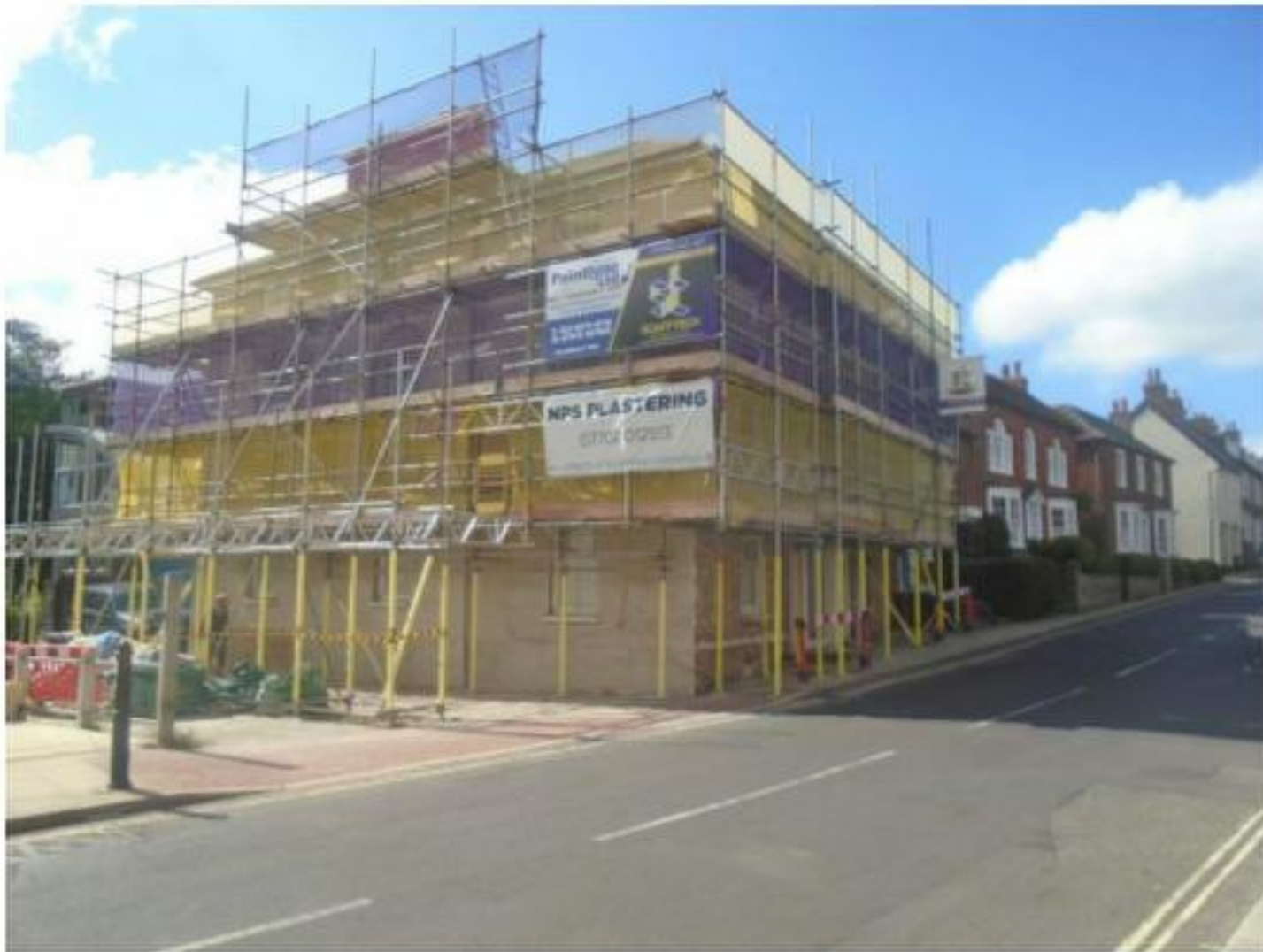
Figure 5. 23 Queen Street (listed building) to west of application site.
