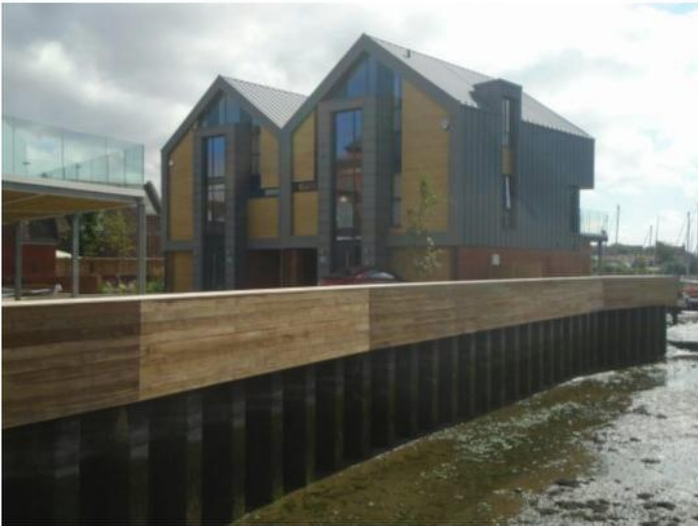
Figure 3. Contemporary style housing to south-east of application site.
