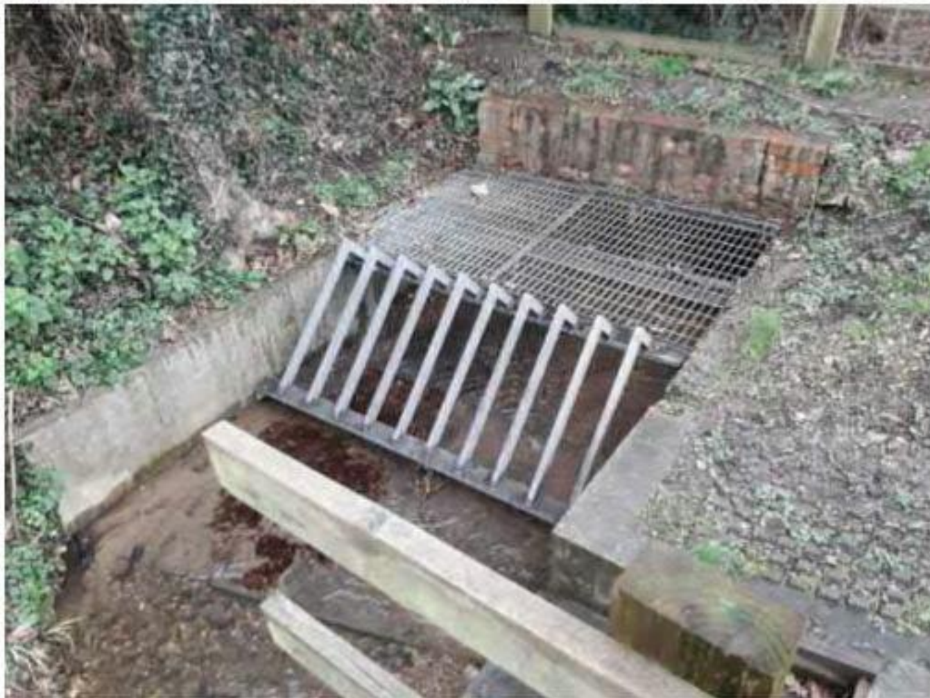
Figure 2 – Watercourse Culvert Inlet adjacent to Portsdown View (Watercourse culverted underground)
