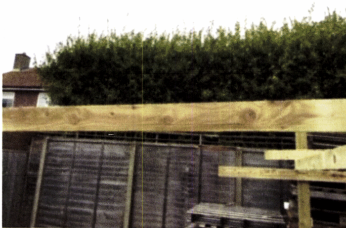
Timber for bike stores & carport.
