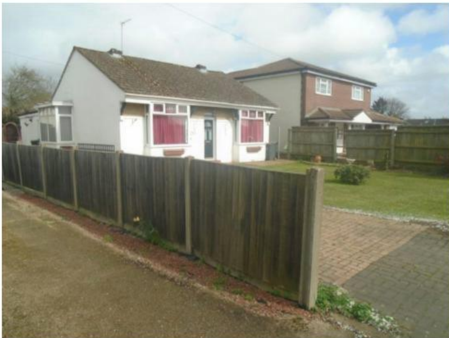
Figure 3. Neighbouring dwelling, No.72.
