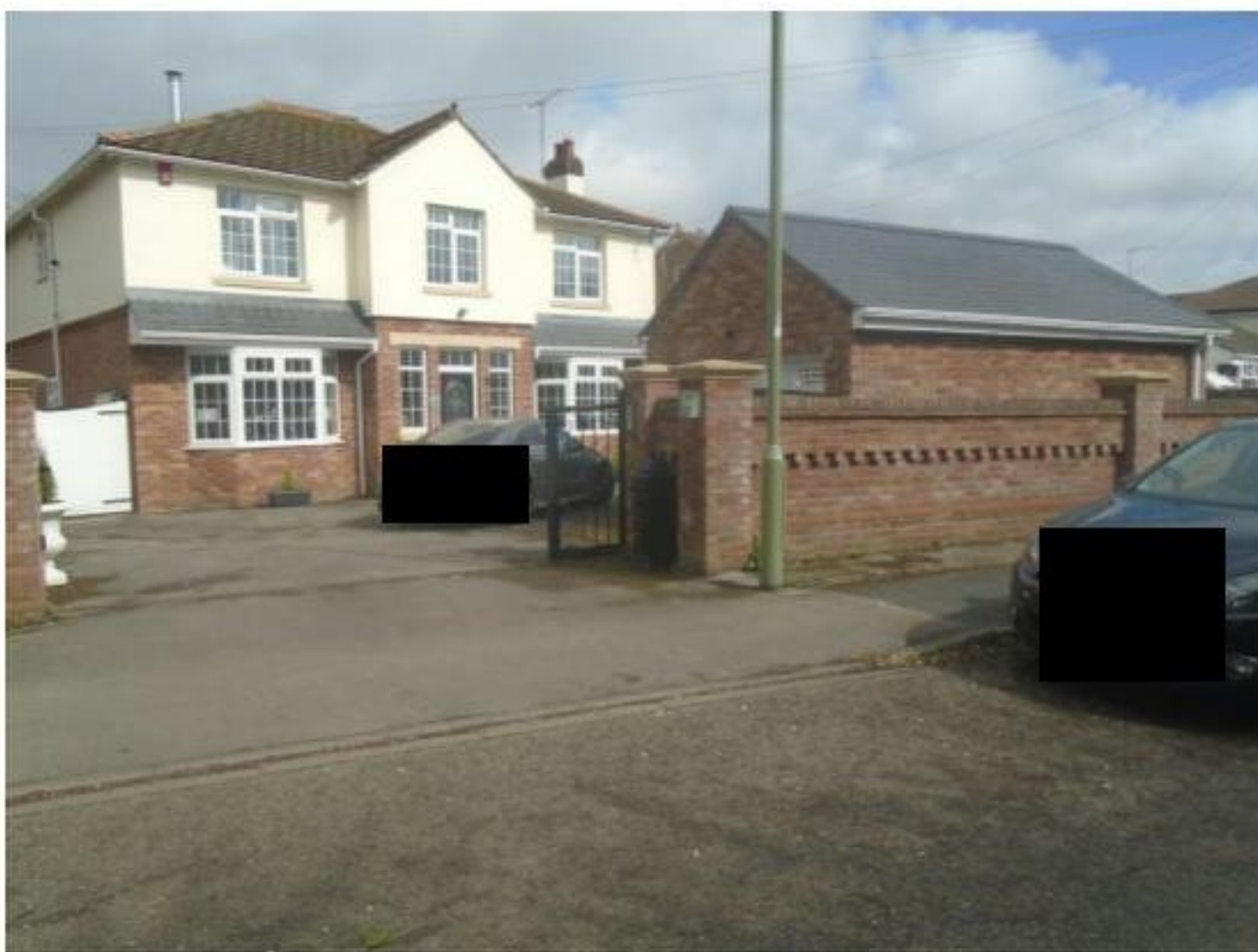
Figure 4. Neighbouring dwelling, No.76.
