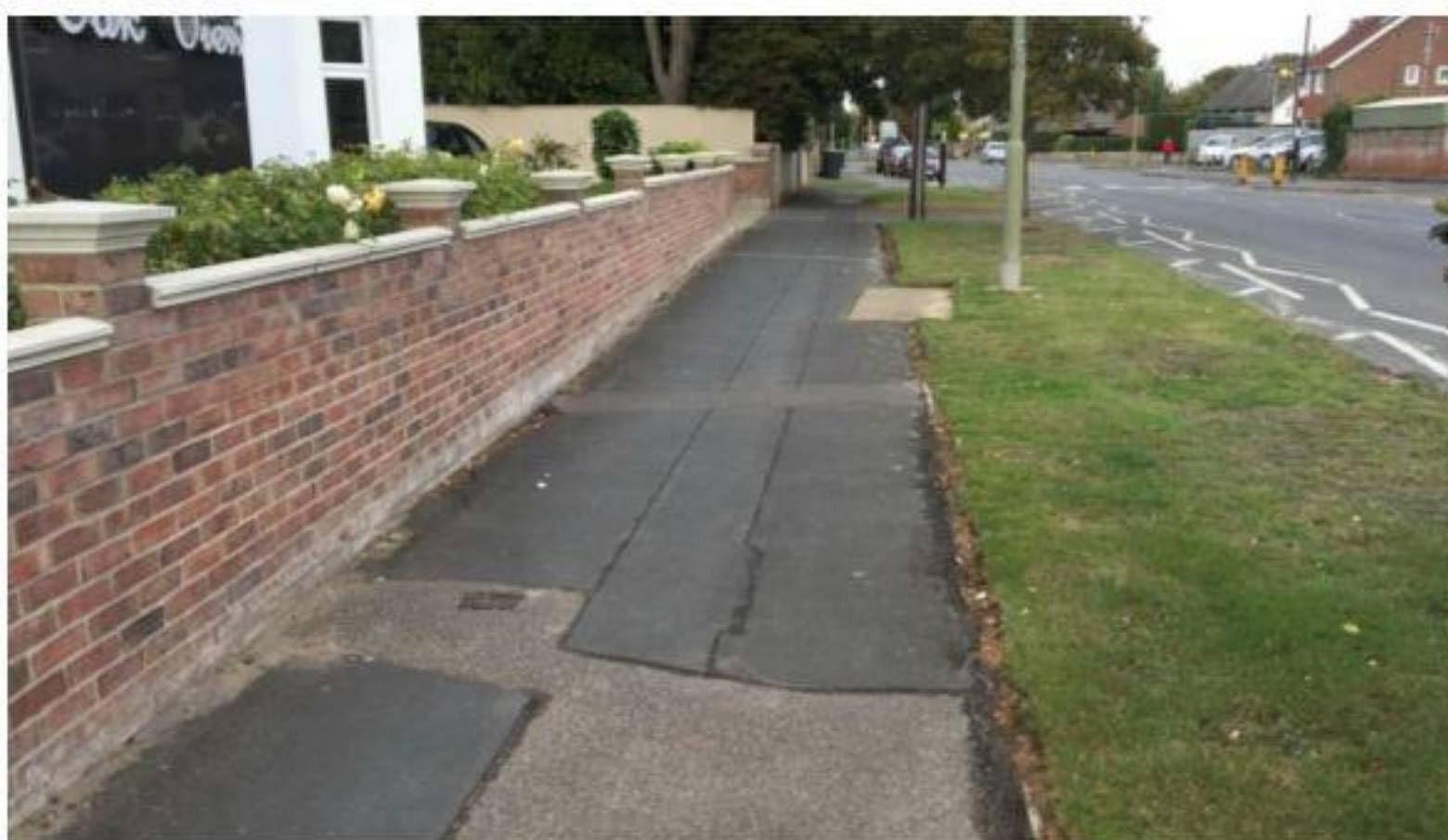
Footway Flanking Beach Road
