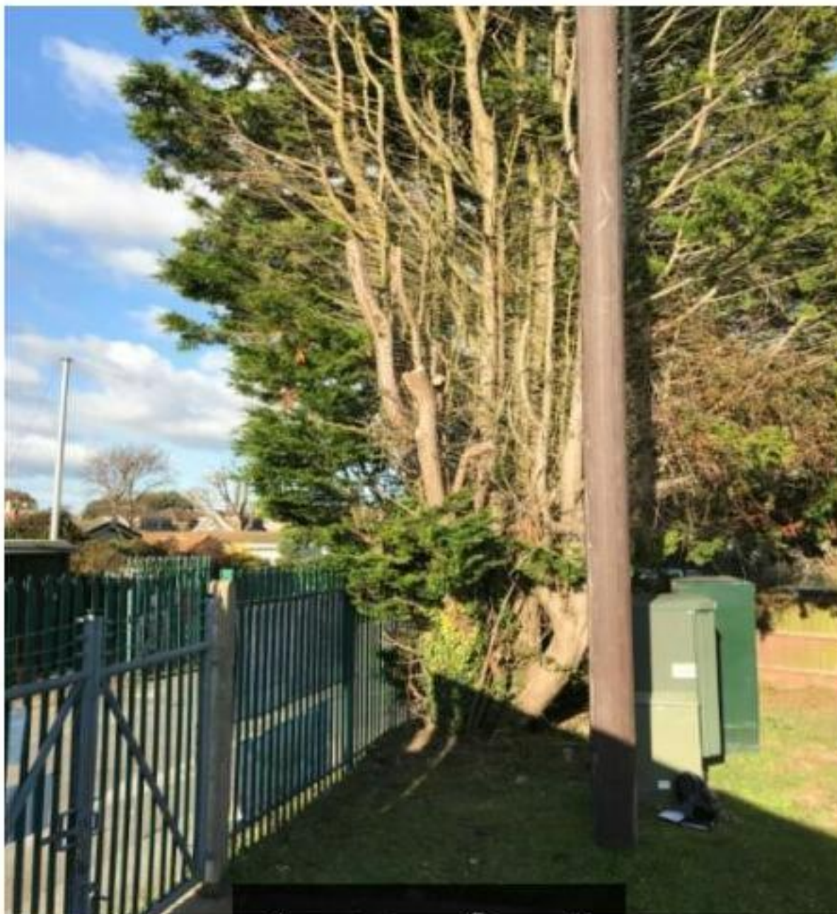
Photograph of cut back to tree to allow for new replacement 15m mast to be installed, note limited space between tree and palisade boundary fence, also note size of base of tree in region of 10-11m high.
