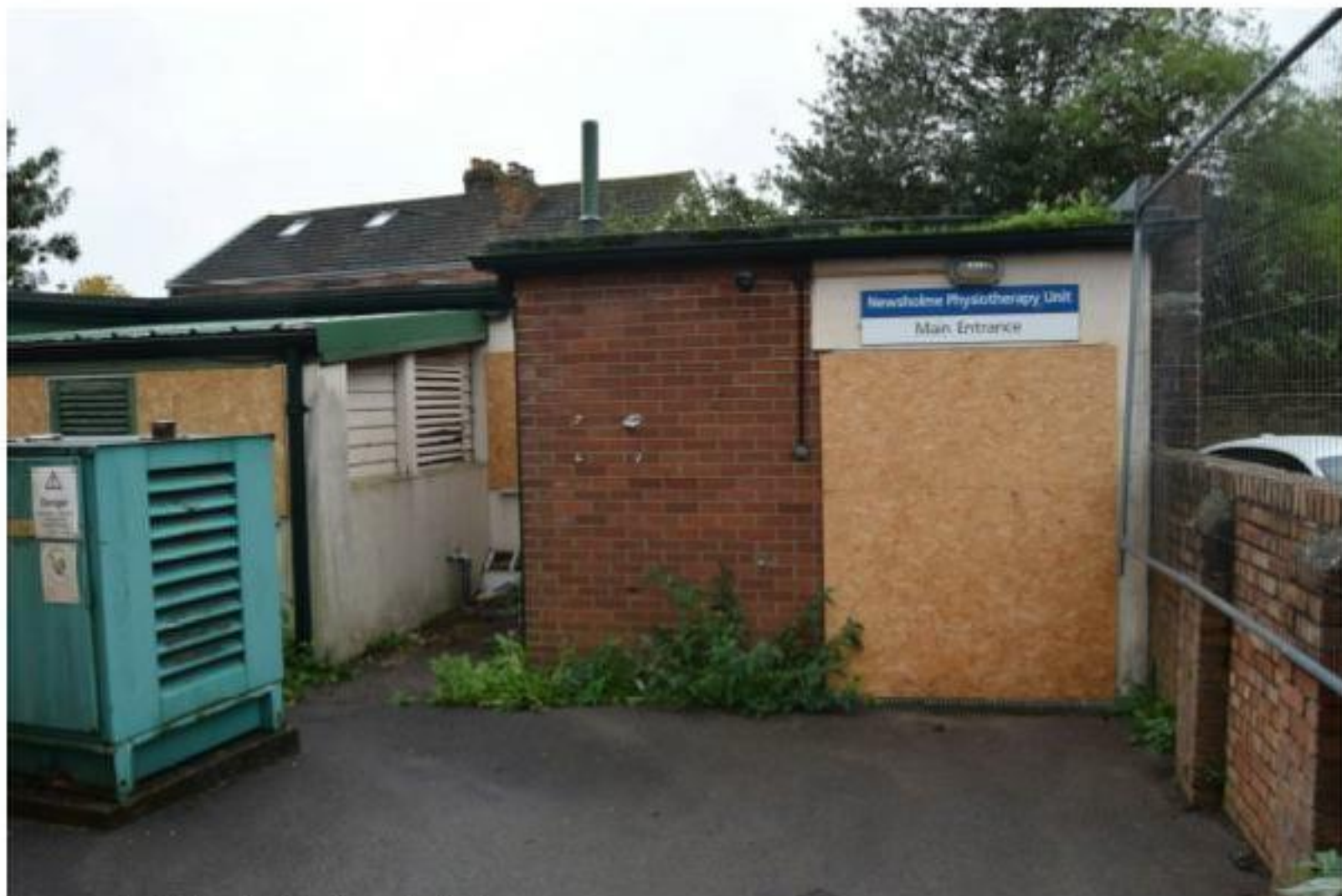
Rear outbuildings (to be demolished)
