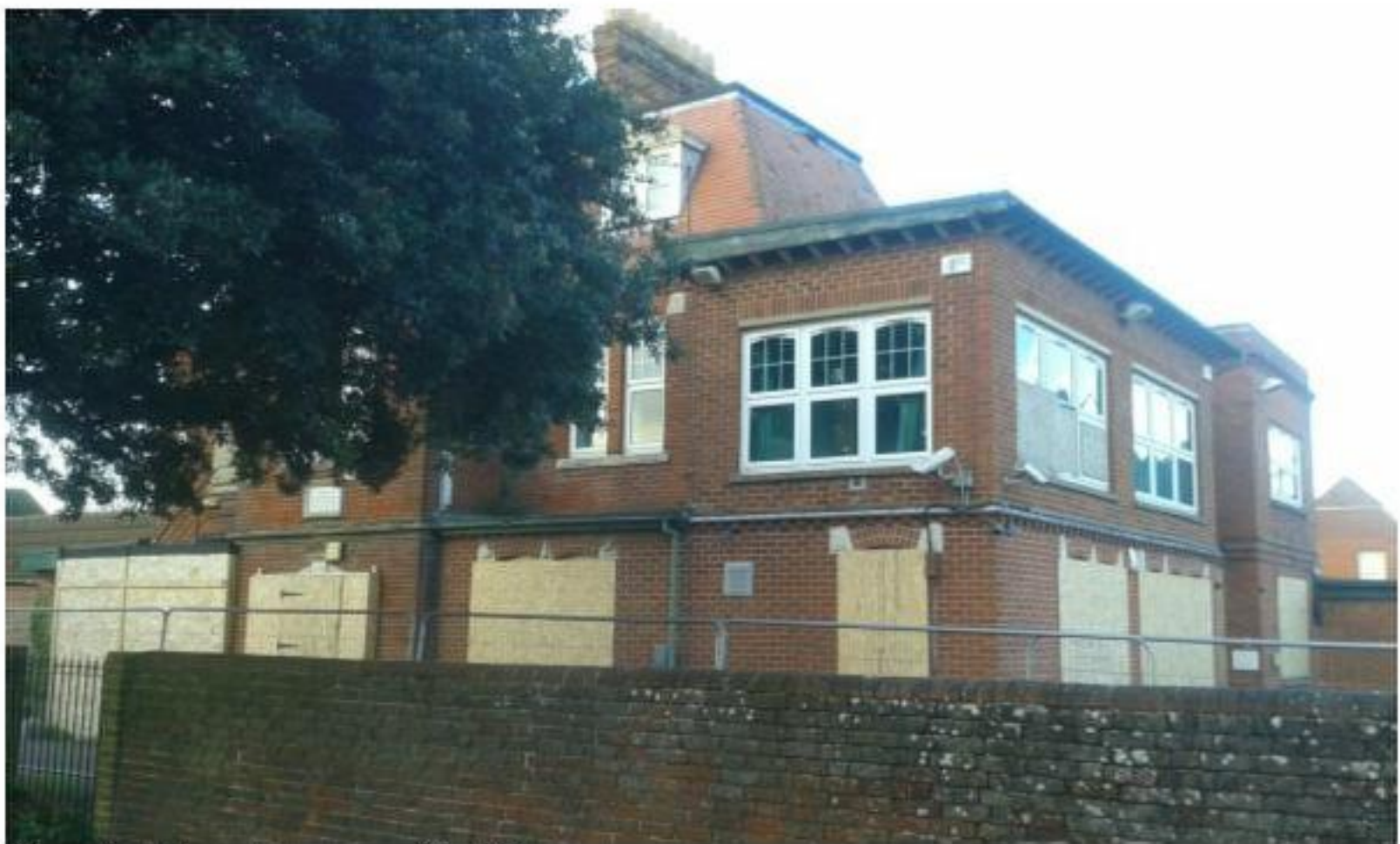
View of south-eastern corner of building
