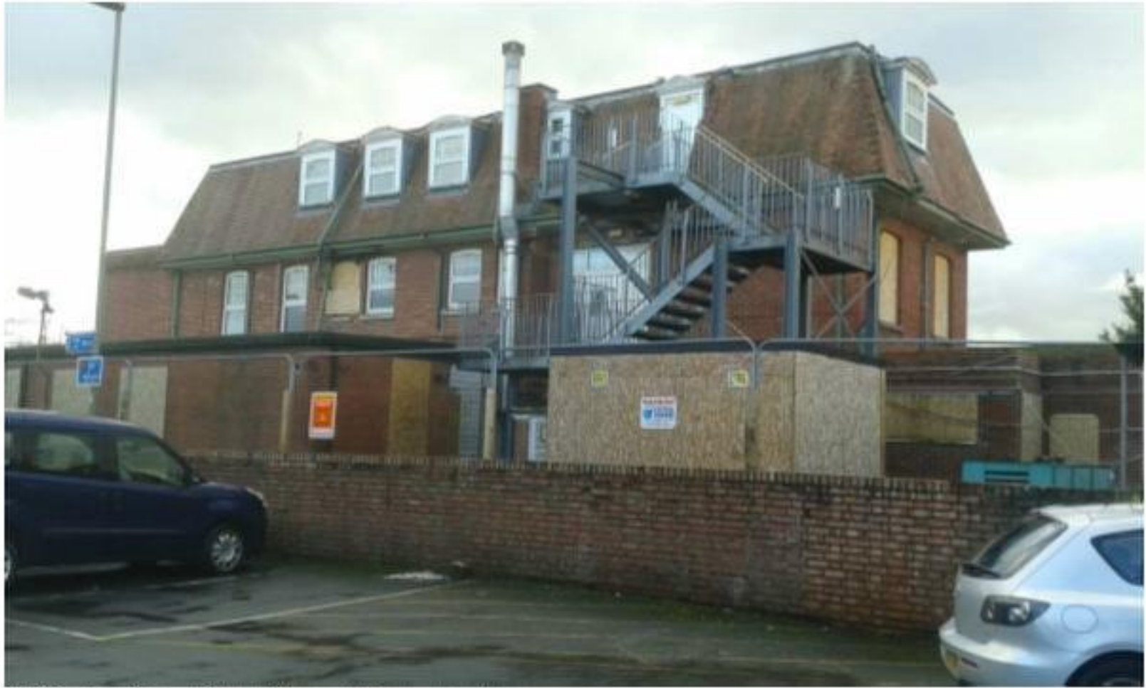
North elevation, viewed from public car park
