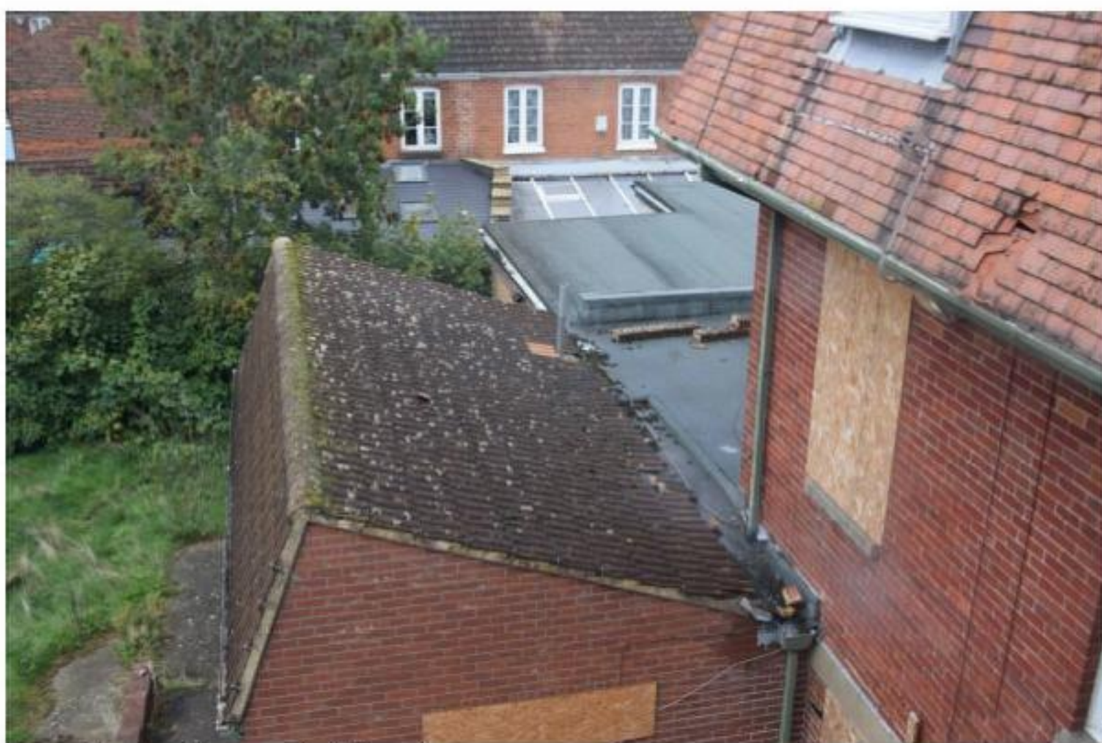
Rear extension with concrete tiled roof
