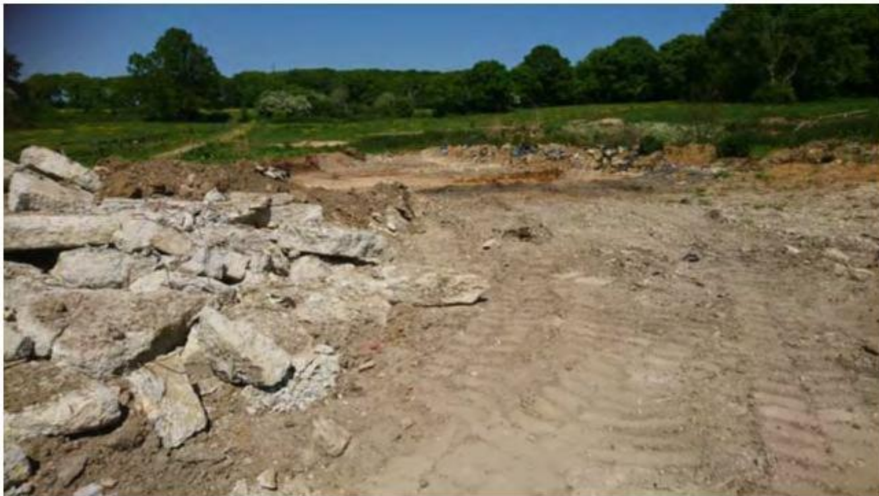
Plate 5 View north of former farmyard area
