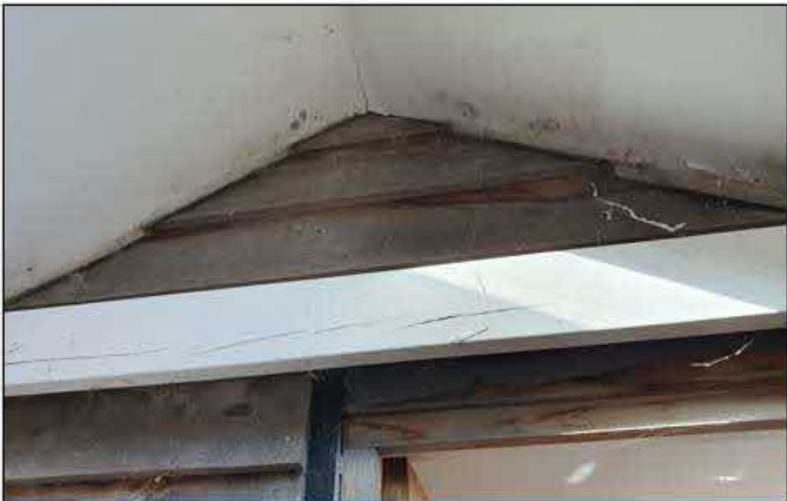
Internal detail of abutment to barn
