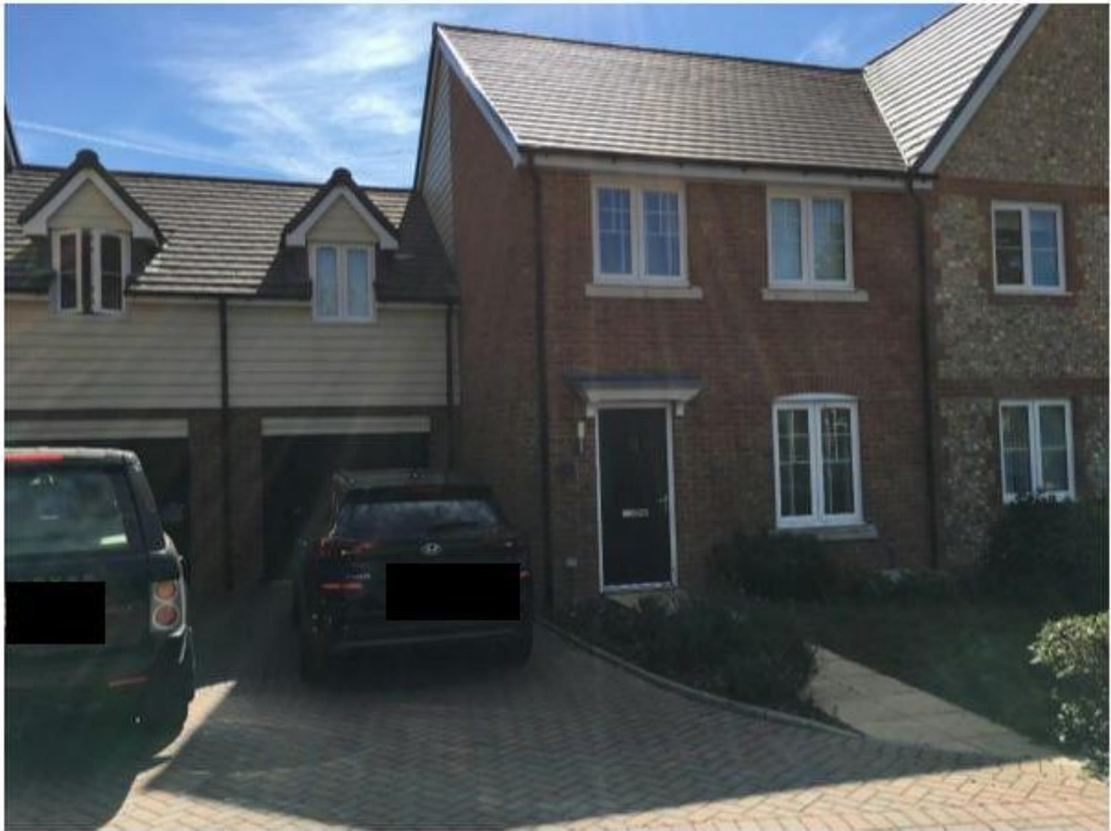
Photo 4: Front of property
