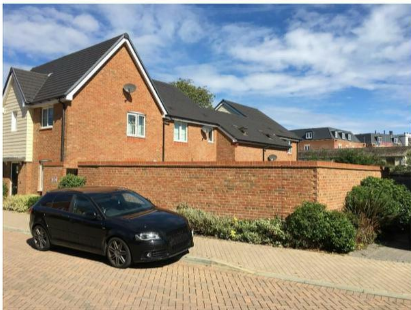
Photo 3: View from street
