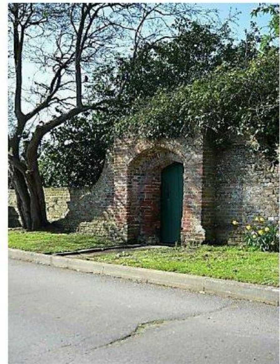
Access permits only light vehicular traffic
