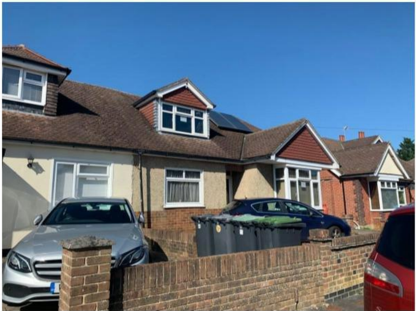
Photo 2: Front East side
