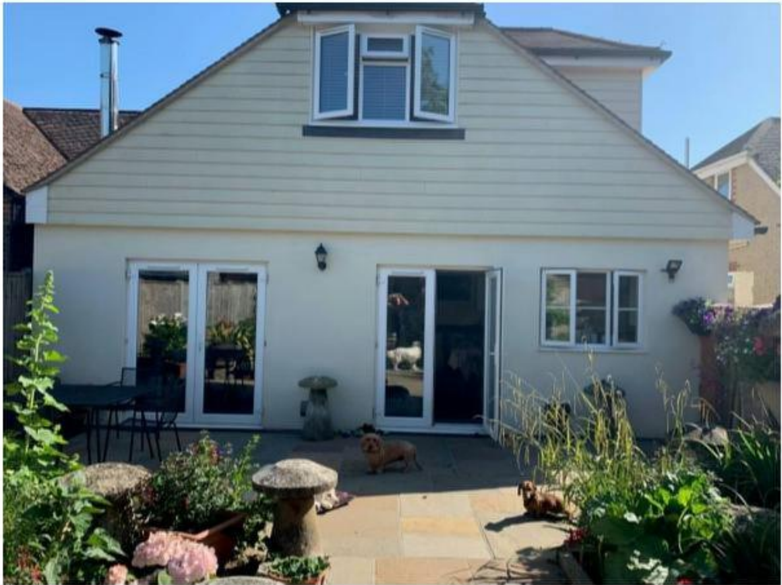
Photo 8: Rear where extension would be
