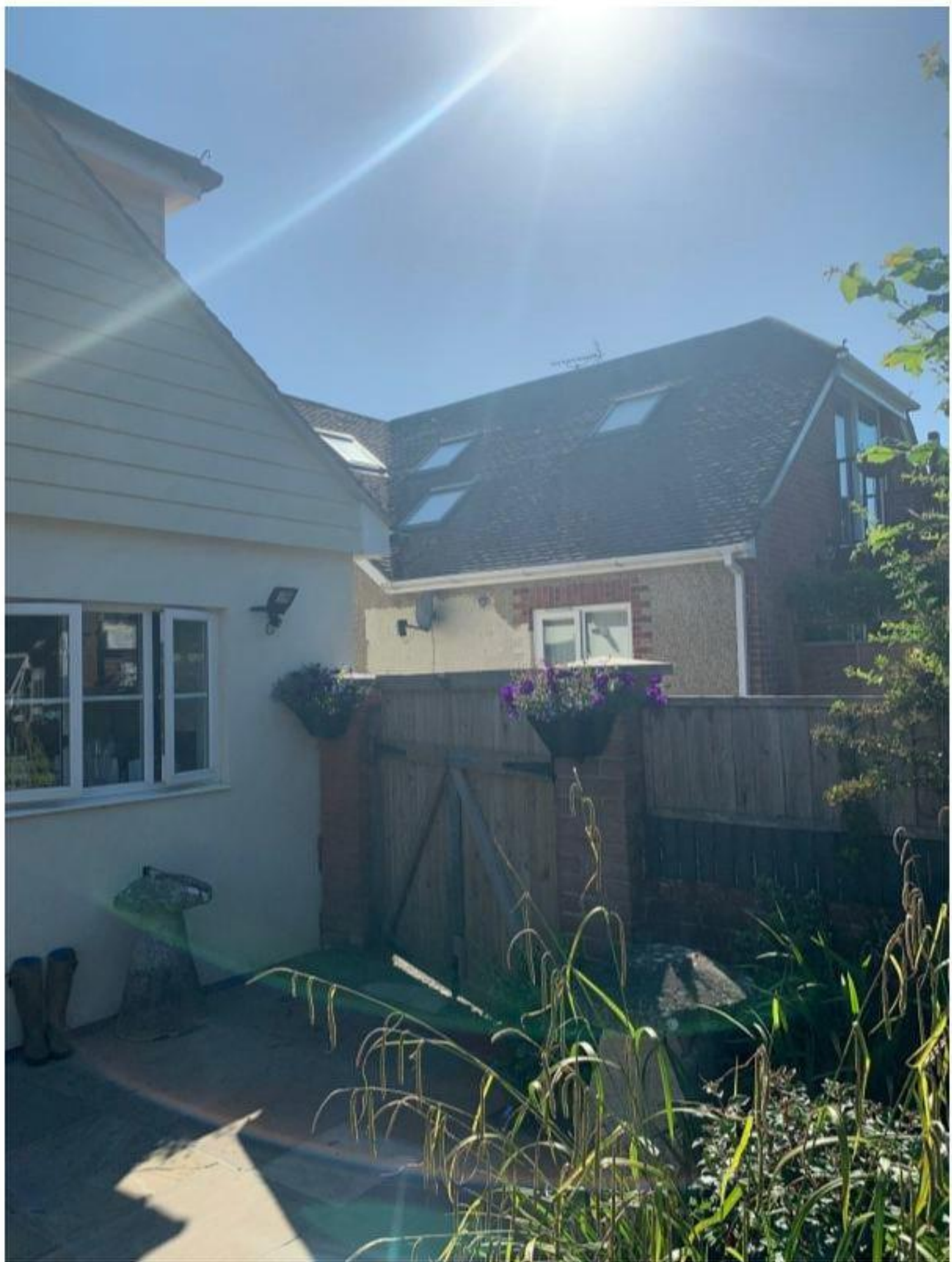
Photo 9: Rear West side
