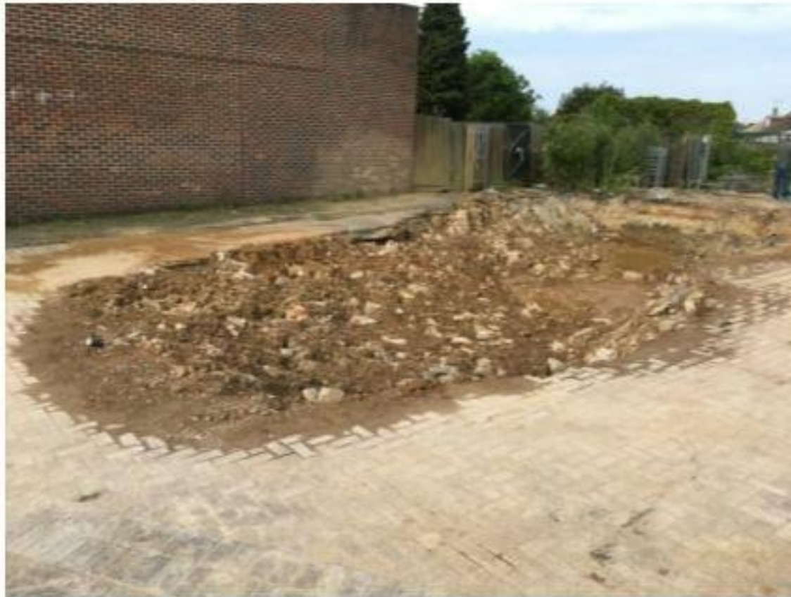
Photograph 1: View of tank excavation, looking south-west.
