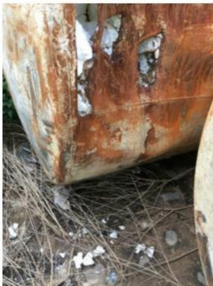
Photograph 4: Inspection of tank, filled with foam.
