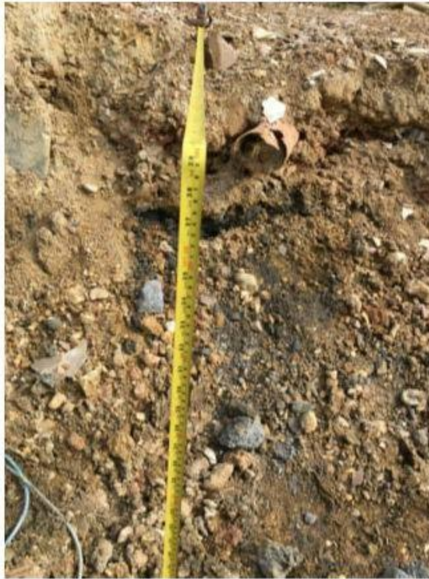
Photograph 9: Depth of the pit at the north-western extent (1.00m).
