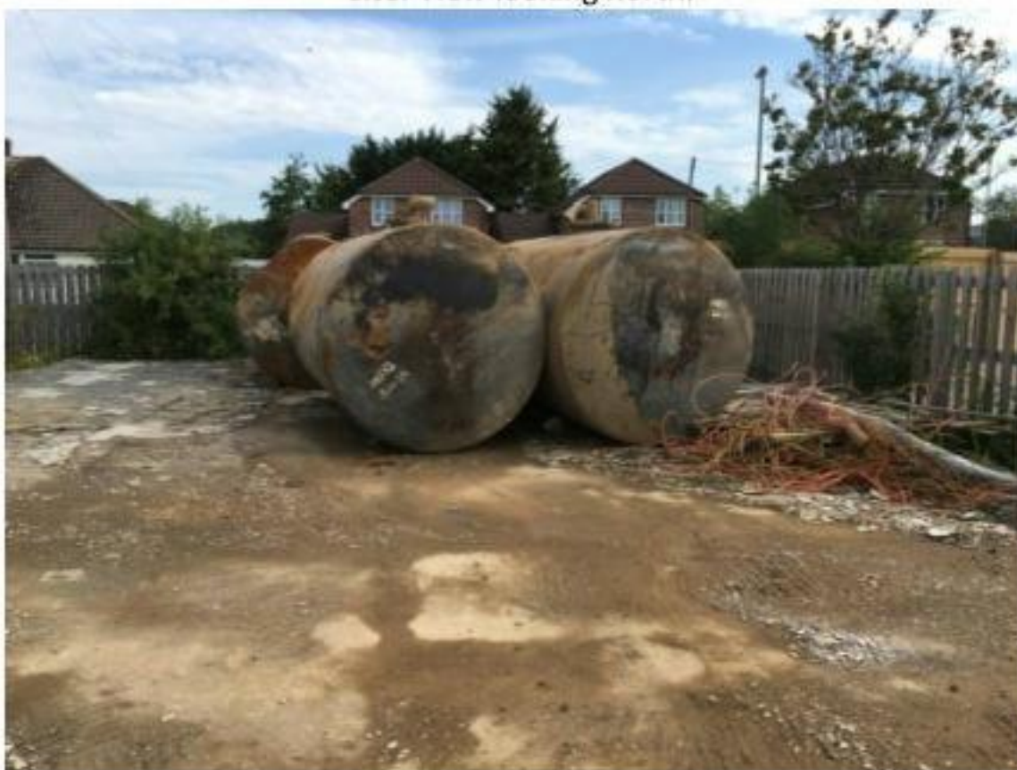
Photograph 3: View of the tanks that had been excavated from the ground, located in the north-west of the site. View looking north.
