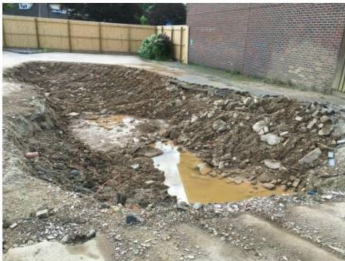
Photograph 2: View of tank excavation, looking south-east.
