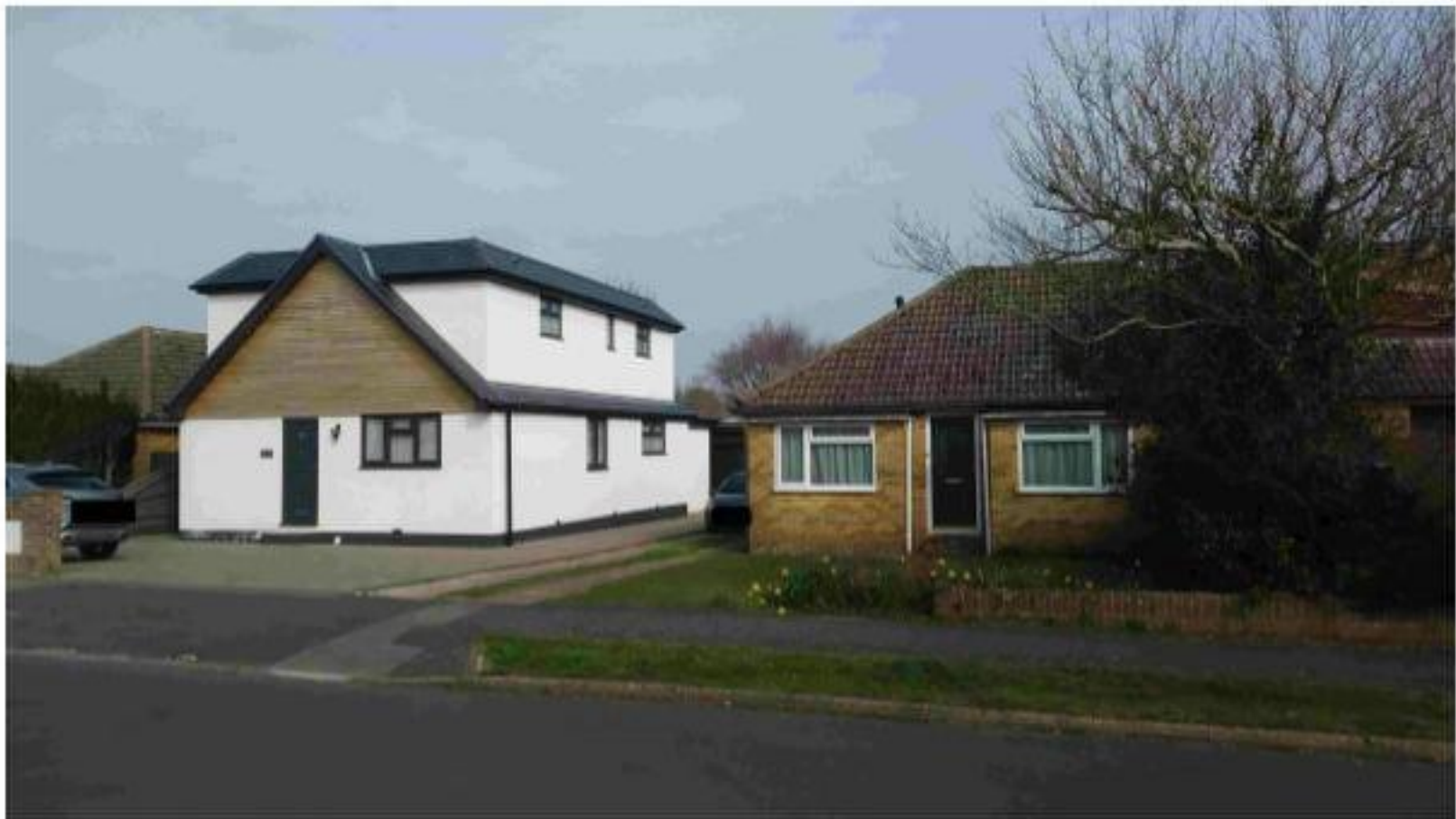
Location 2 – 135 Silverdale Drive
