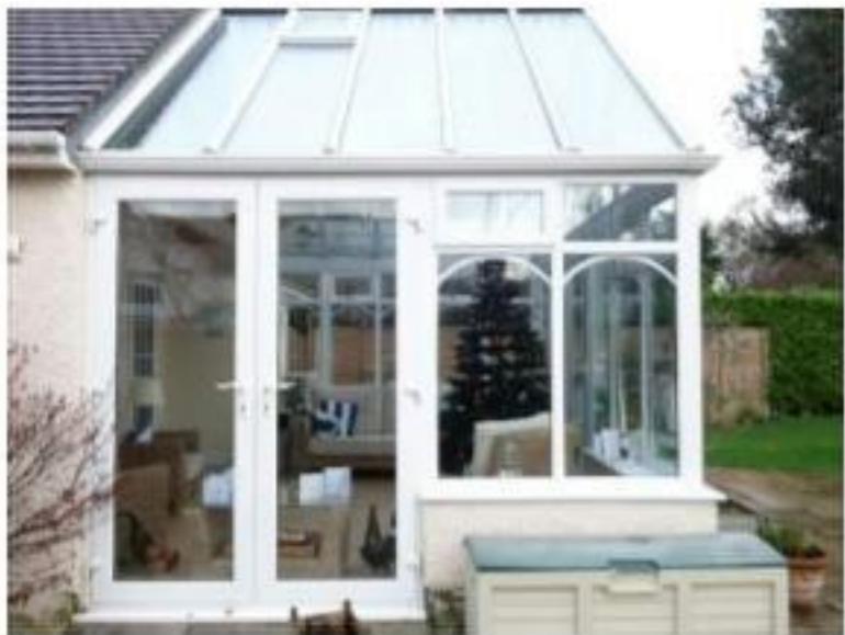
(G). Side elevation image of conservatory at #61, side/rear access door, that will be affected by the proposed scheme with the loss of privacy and over dominant structure.
