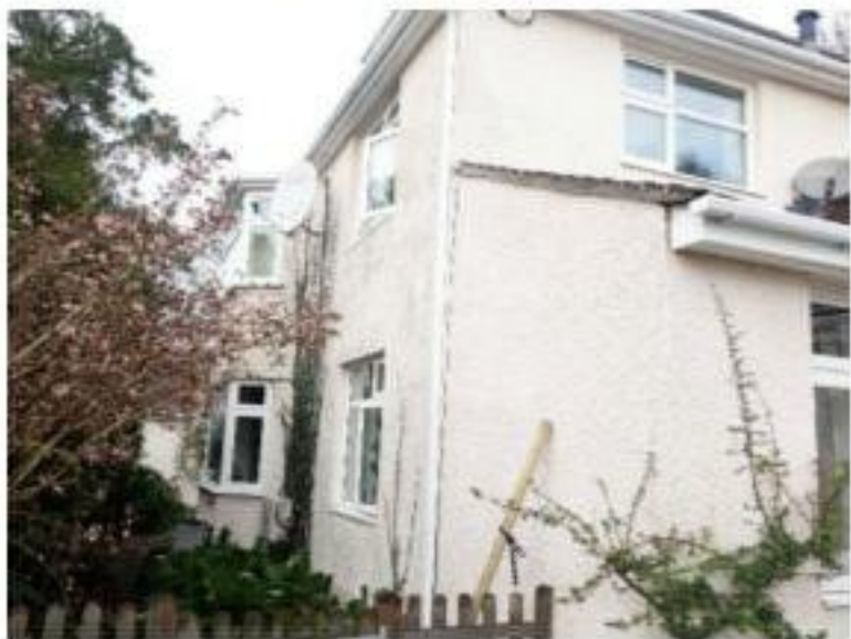
(H). Side elevation image of #61, showing the ground and first floor windows, rear access, that will be affected by the proposed scheme with a loss of privacy and over dominant structure.
