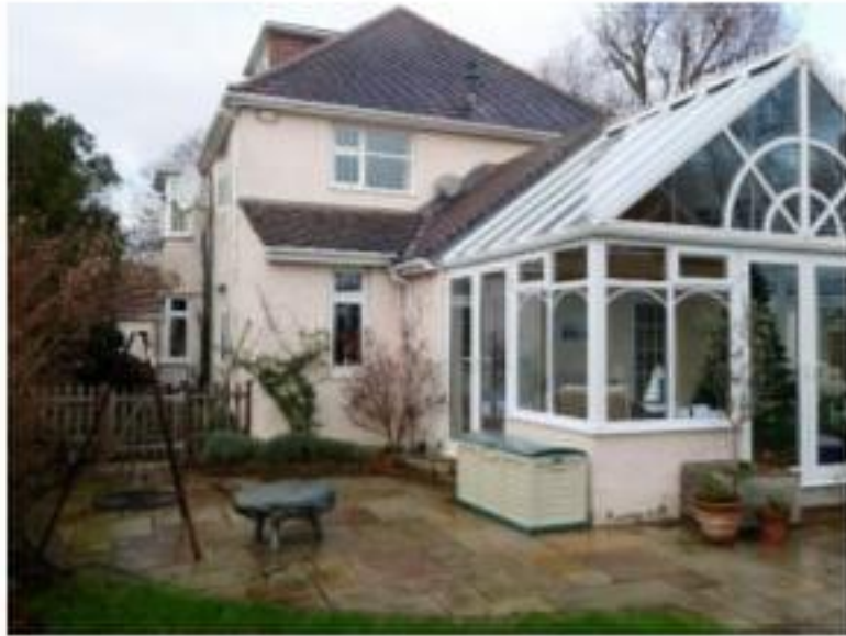
(F). Side elevation image of #61 showing the ground and first floor windows, conservatory, rear access doors and patio private amenity area, that will be affected by the proposed scheme with a loss of privacy and over dominant structure.
