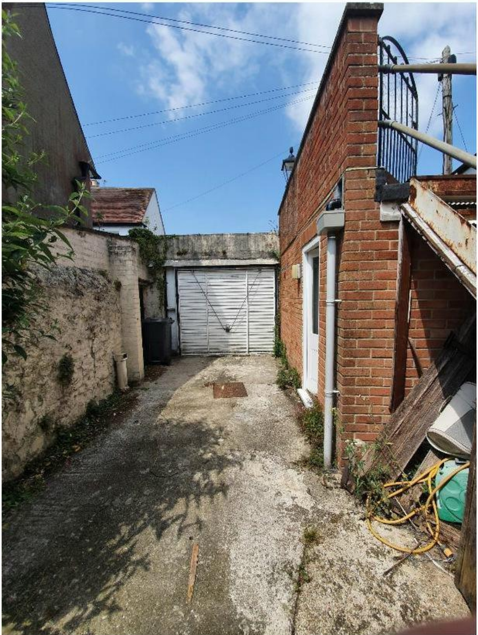
This photograph shows the garage door in place (now removed for safety reasons)
