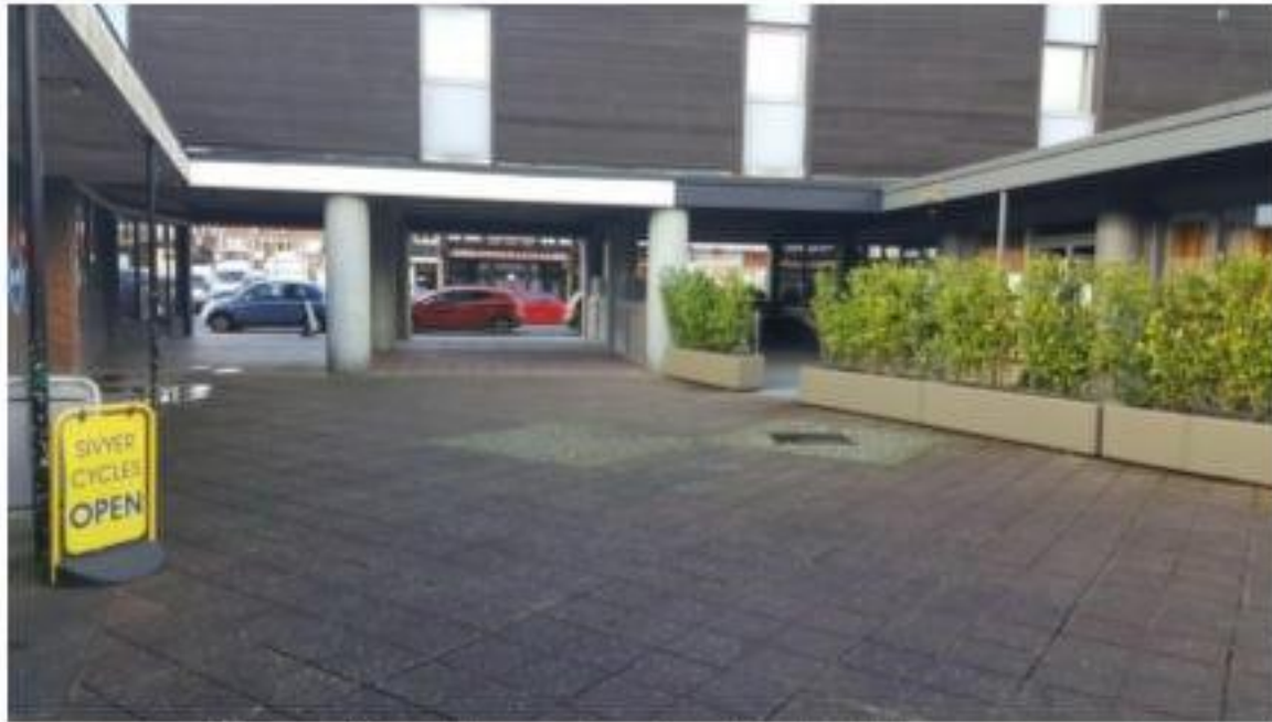
Photograph 2: Existing Undercroft Pedestrian Walkway
