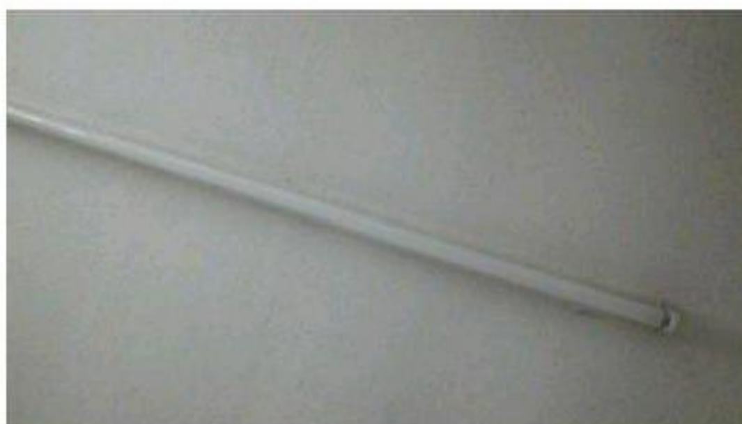
Sample 31: House Building. First Floor. Room 2. Artex coating to plasterboard ceiling
