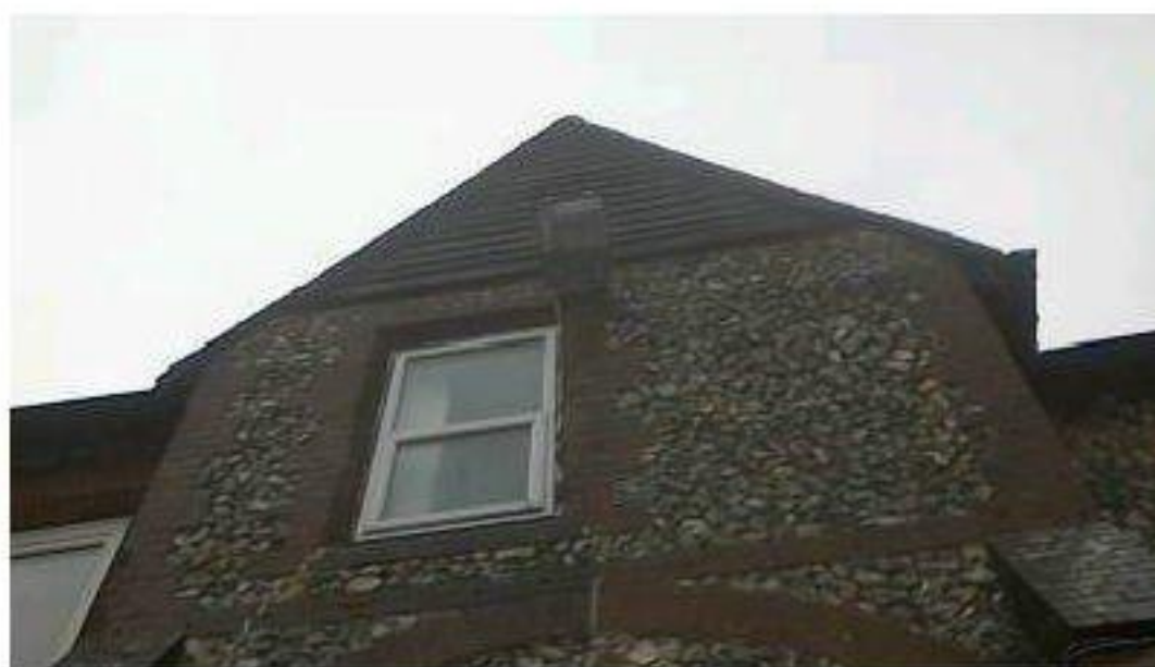
Visual 1: House Building. First Floor. External. Cement undercloaking to high level pitch roofs
