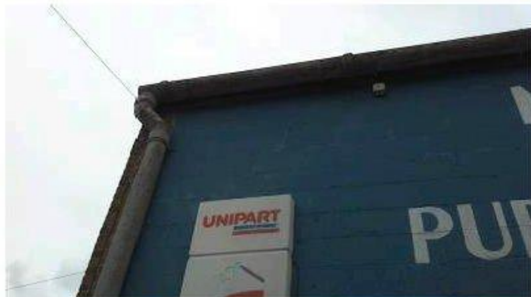
Sample 24: Workshop Building. External. External. Cement downpipe/guttering to east/west sides of bay 4 section
