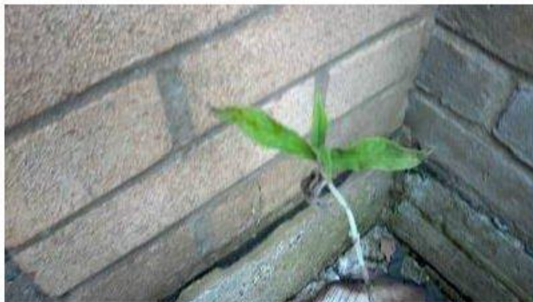
Sample 26: Workshop Building. External. External. Typical damp proof course surrounding building
