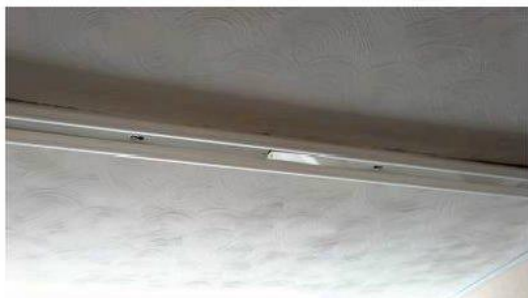
Sample 3: Out Building (Car Sales). Ground Floor. Kitchen. Textured coating to plasterboard ceiling
