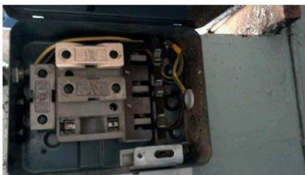
Sample 11: Workshop Building. Ground Floor. Office 1. Woven flash pads within fuse box
