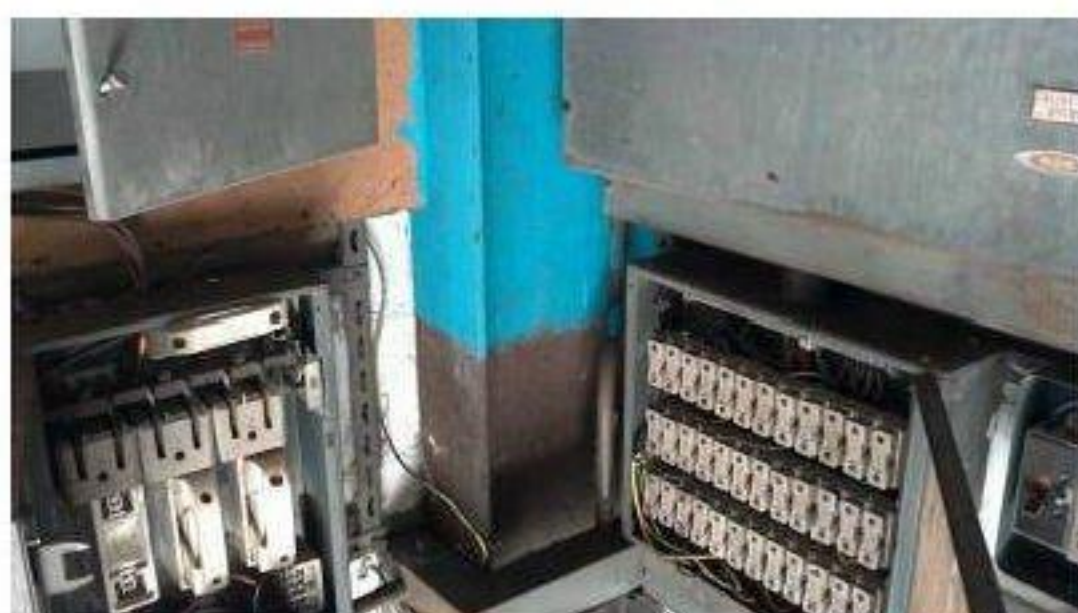
Ref. Sample 11: Workshop Building. Ground Floor. Bay 2. Woven flash pads within fuse boxes to north east corner
