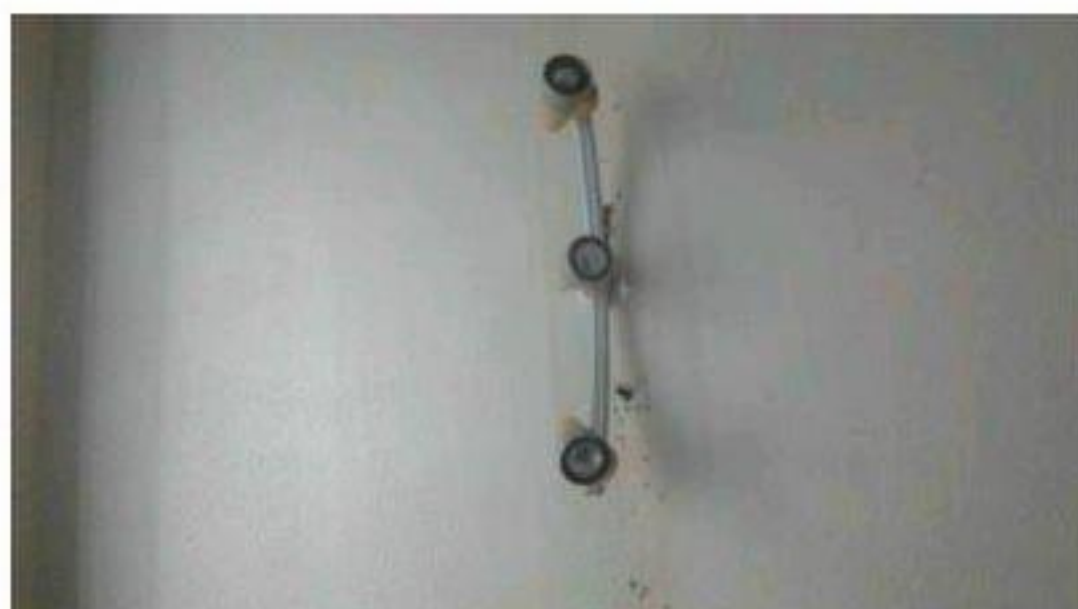
Sample 30: House Building. First Floor. Room 1. Artex coating to plasterboard ceiling
