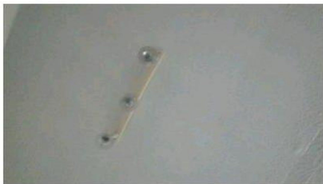
Sample 32: House Building. First Floor. Room 4. Artex coating to plasterboard ceiling
