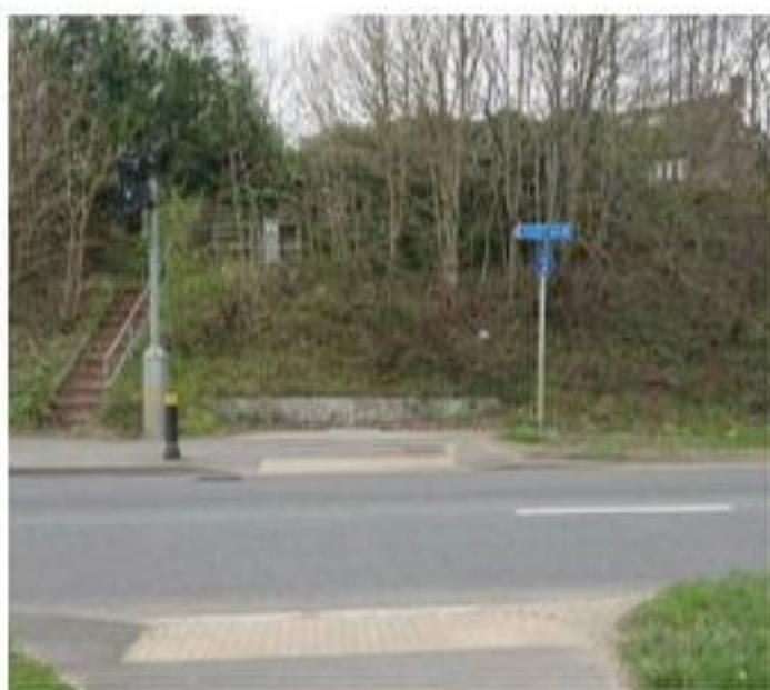
Photograph 4: Pedestrian crossing A3(M) on-slip
