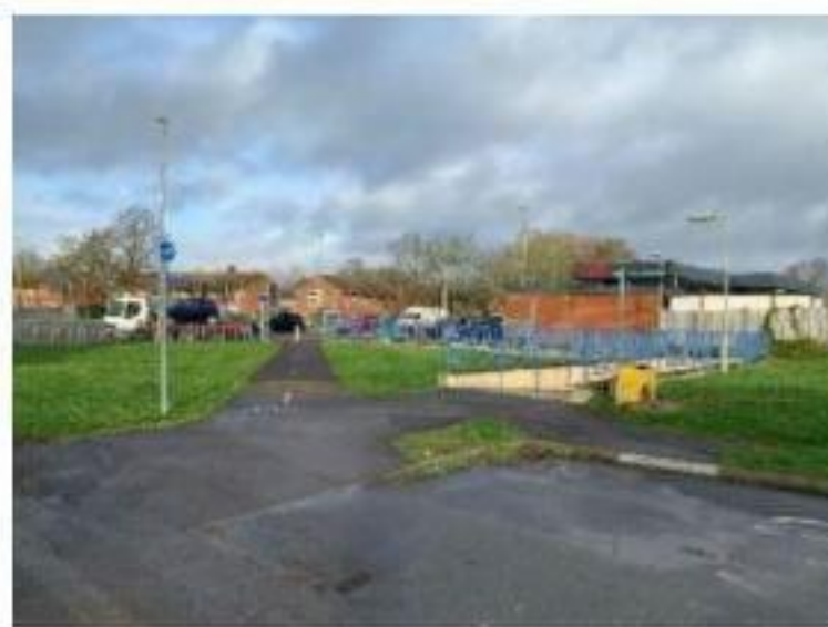
Photograph 2: Petersfield Road Subway
