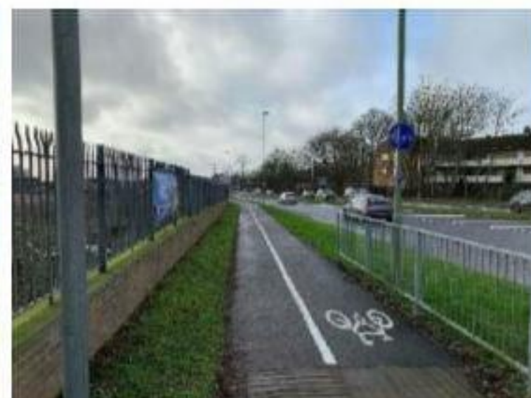
Photograph 4: Route NCN 22 Southbound
