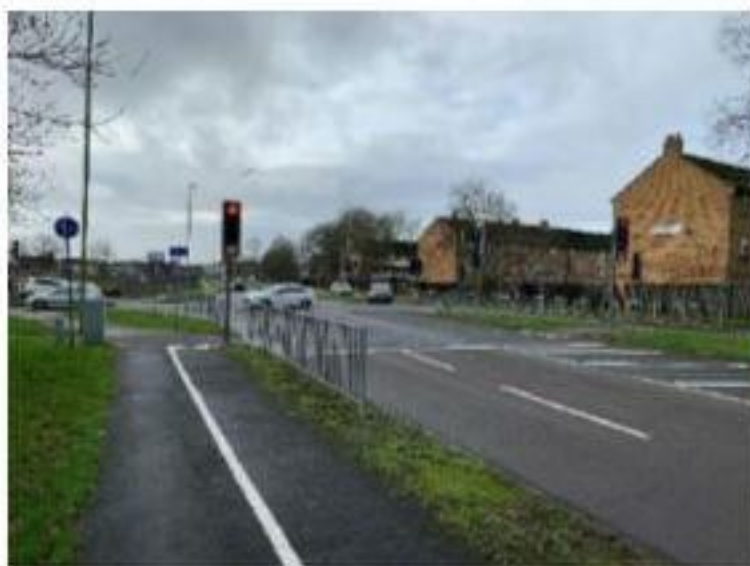
Photograph 1: Petersfield Road Pedestrian Crossing
