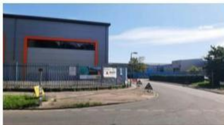
New Lane corner junction with Stanbridge Road
