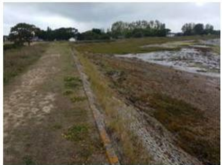
Photo 8: View of the flood embankment looking towards the centre of the Park
