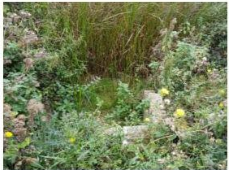
Photo 2: Area no.1 – surface water outfall into the drainage ditch
