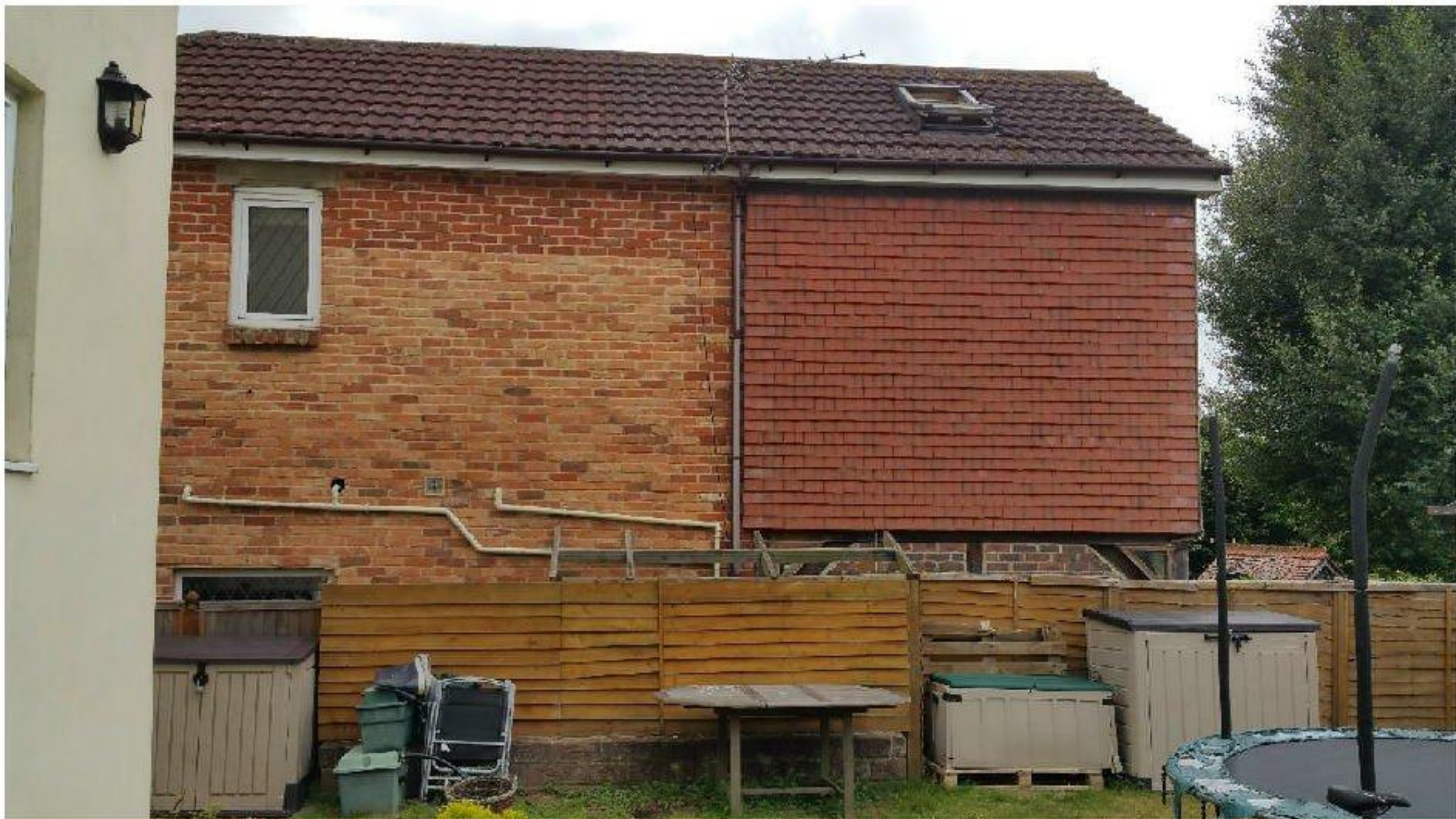
Side view of No15 Lovedean Lane taken from garden of No17 Lovedean Lane facing East. It can be seen how far the two-storey extension extends past No17 blocking garden in completely.
