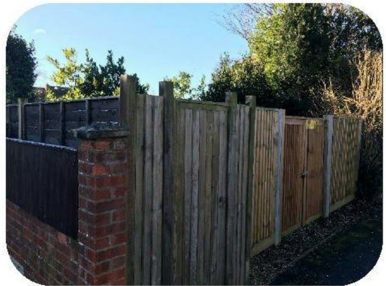
Hallett Rd Sub-Station
