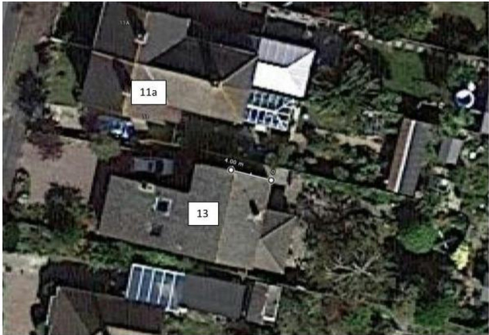
Difference between existing building line at 11a and 13 Mengham Avenue
