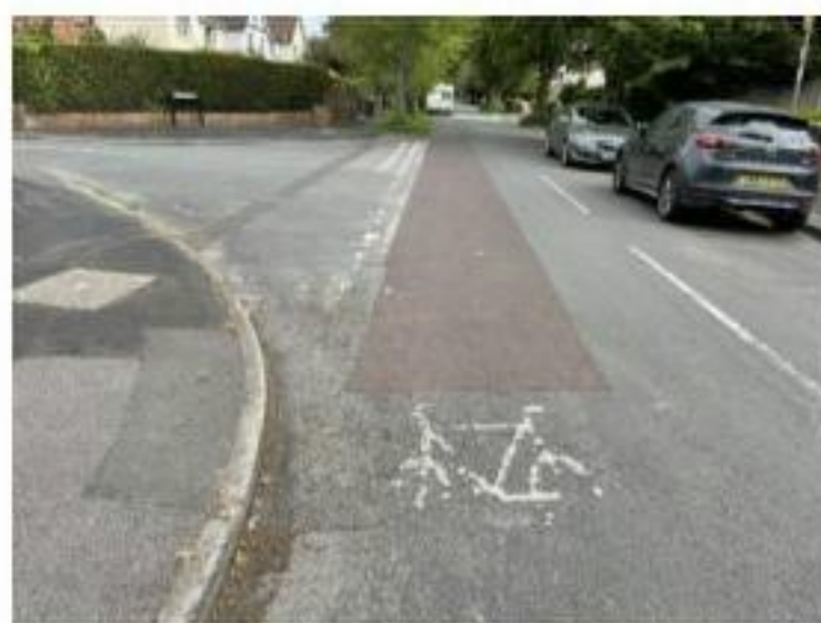
Photograph 9: Road Markings across Castle Avenue / Castleway Junction
