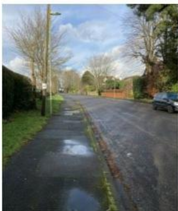
Photograph 6: Existing Footways along Warblington Avenue
