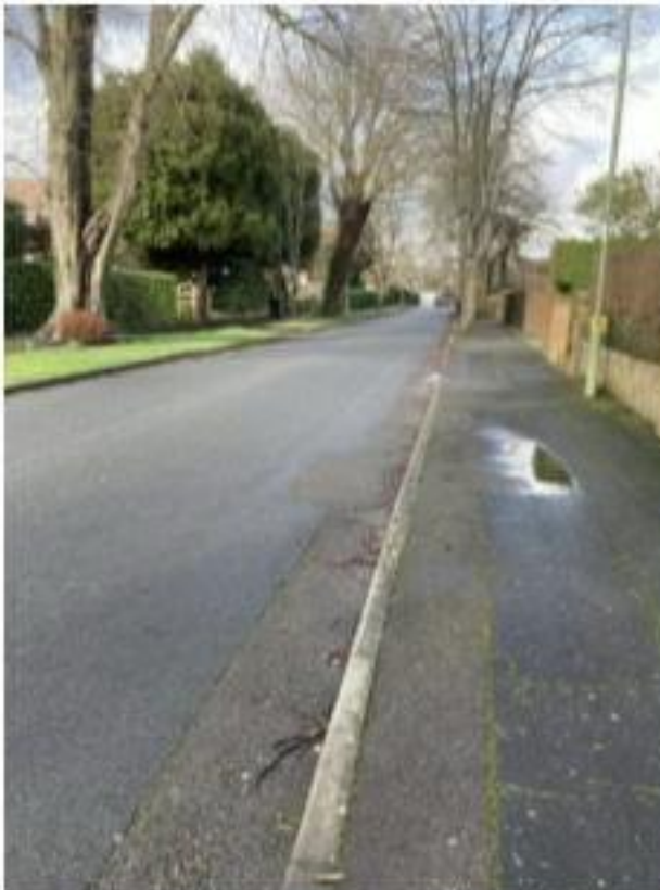
Photograph 6: Footways along eastern side of Castle Avenue (towards the site)
