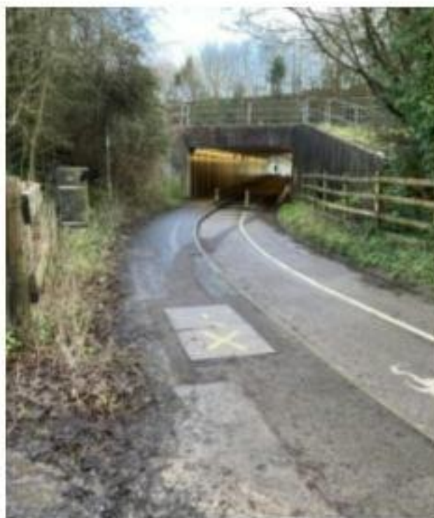
Photograph 21: Entrance to A27 Subway from Emsworth Road
