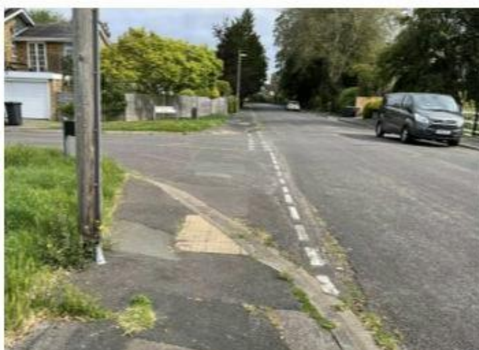
Photograph 7: Tactile Paving Crossing across Warblington Avenue / Woodpecker Close junction
