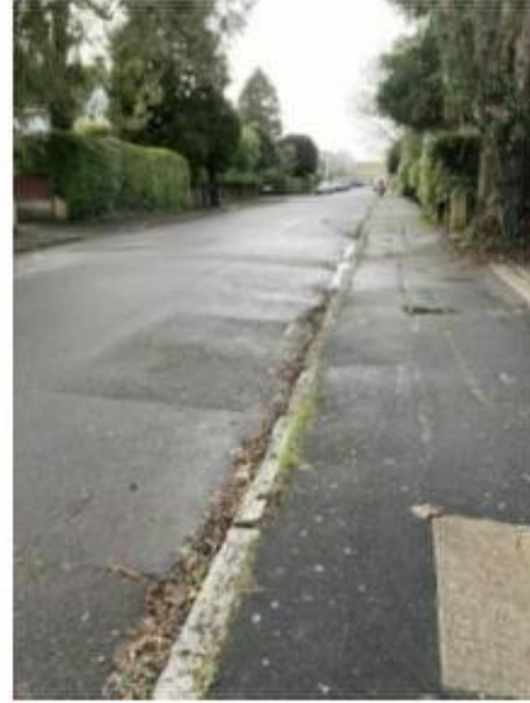
Photograph 3: Footways along St George's Avenue (towards Southleigh Road)
