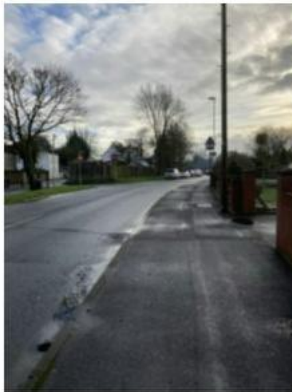
Photograph 9: Footways along Western Side of Southleigh Road
