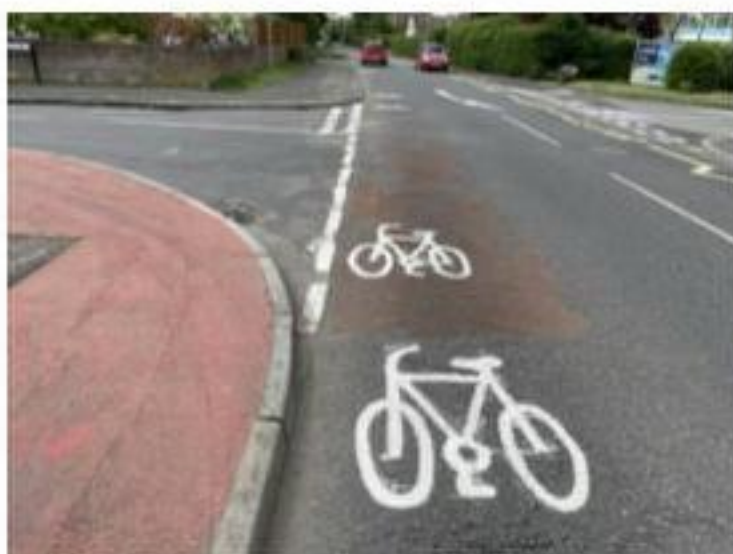
Photograph 15: Cycle Markings at Southleigh Road / St George's Avenue junction
