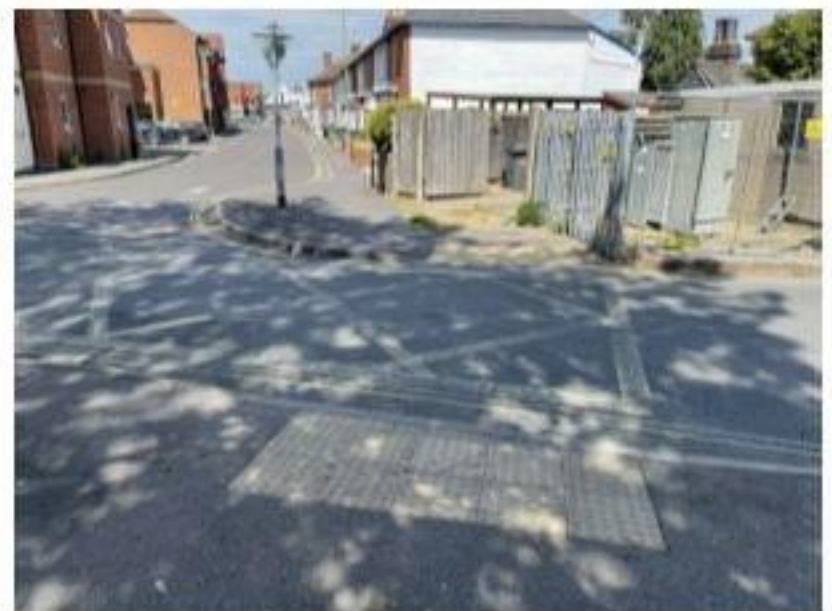
Photograph 20: Crossing on New Lane (north of Waterloo Road)
