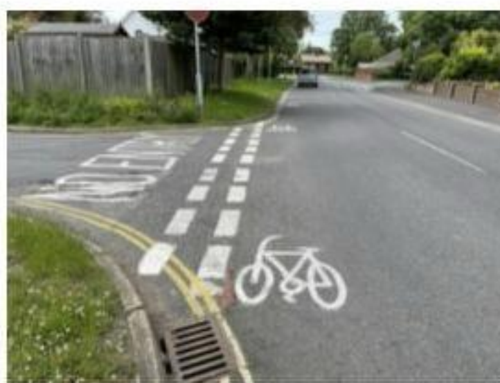
Photograph 14: Cycle Markings at Southleigh Road / Southleigh Road junction
