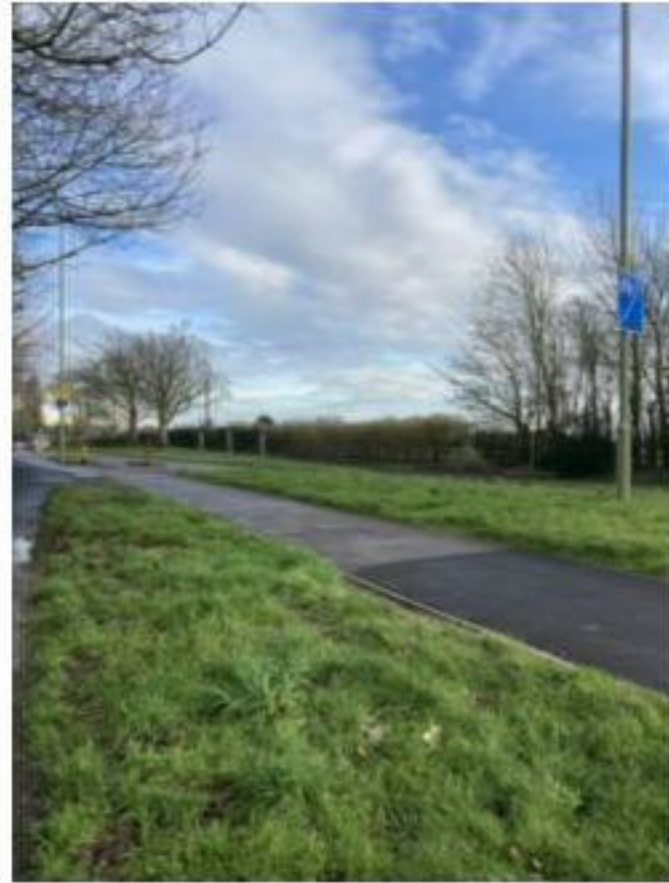
Photograph 238: Footway along Havant Road
