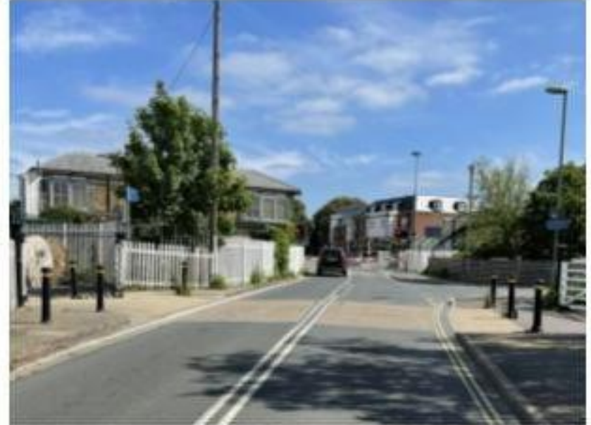
Photograph 26: Pedestrian Crossing on New Lane
