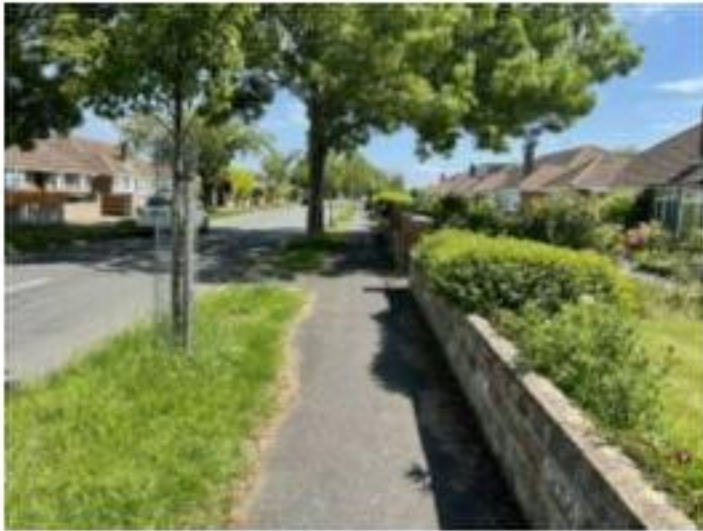
Photograph 27: Existing Footways along Selangor Avenue
