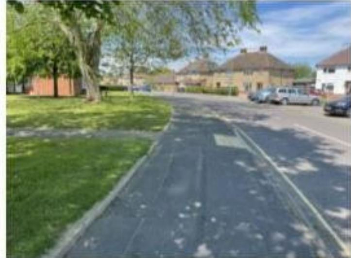
Photograph 28: Existing Footways along Victoria Road
