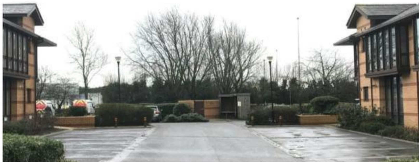
Figure 3 View of Application Site from North-West
