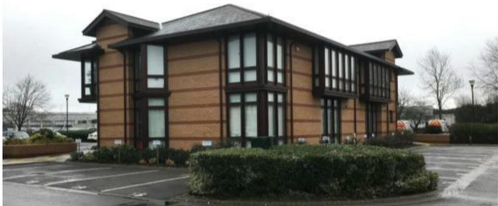
Figure 11 Typical Existing Office Building within The Briars
