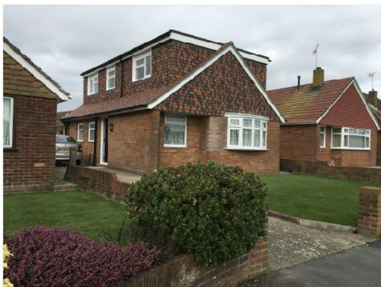
The west elevation of the subject dwelling.
