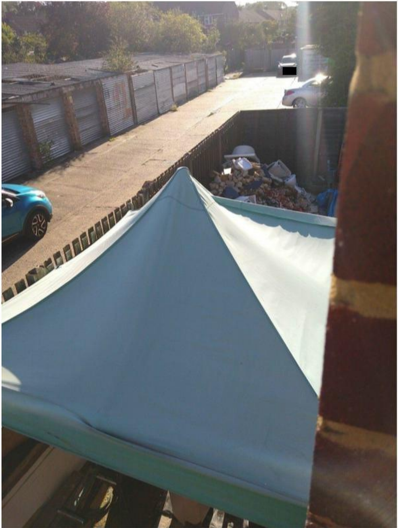
Photo 7: First floor rear view
