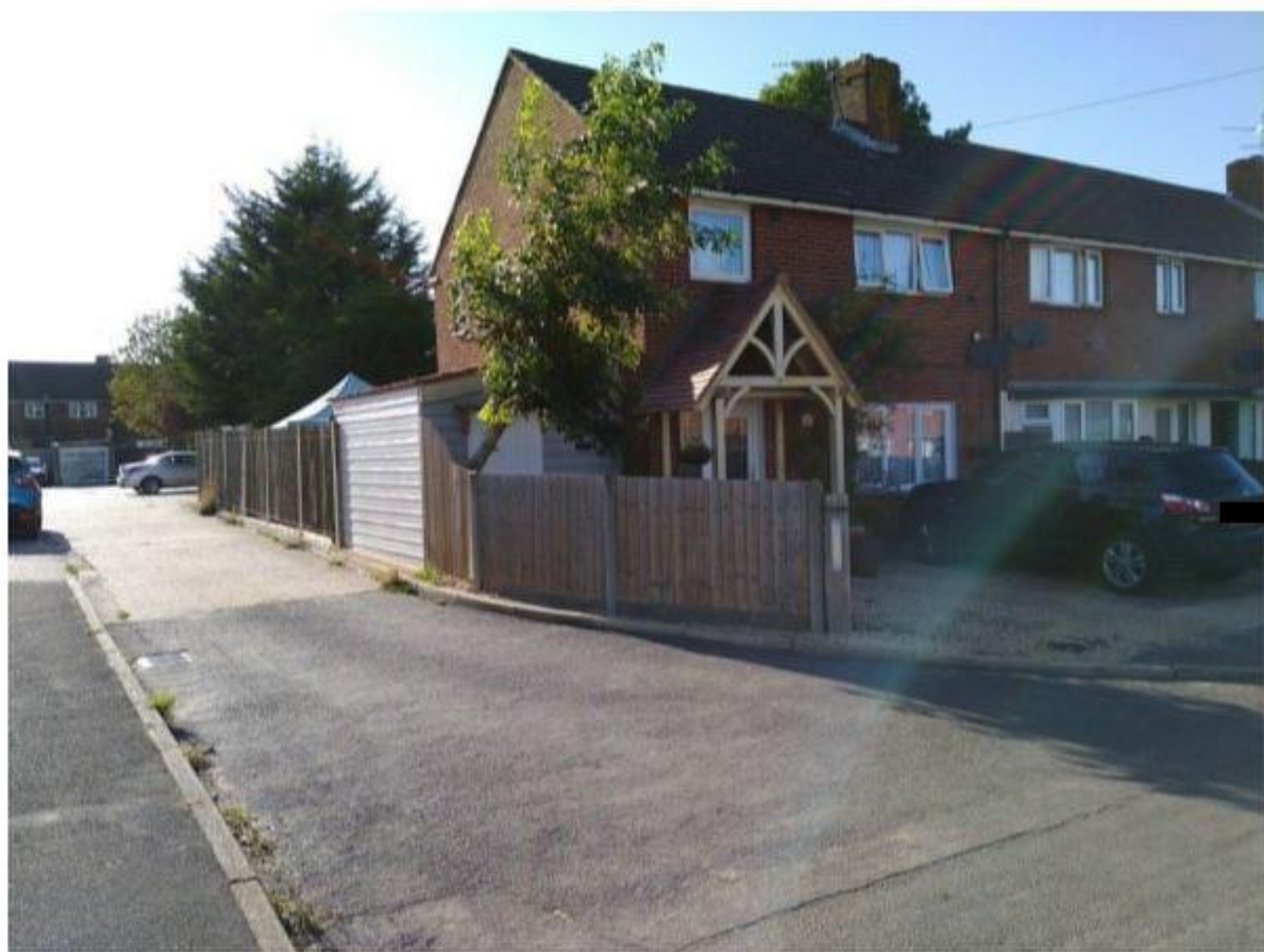
Photo 4: Front/side of the property
