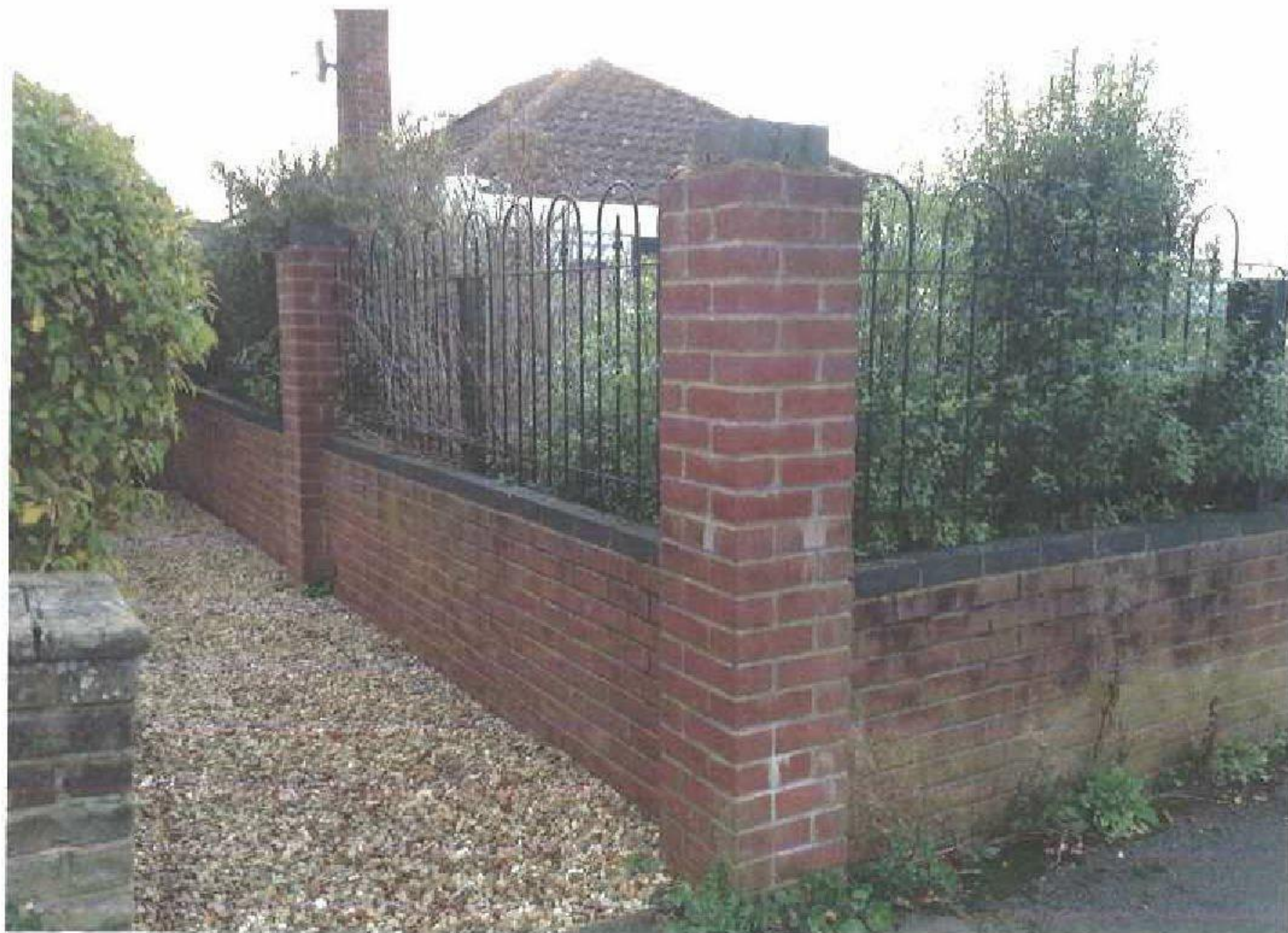
North East corner of property
