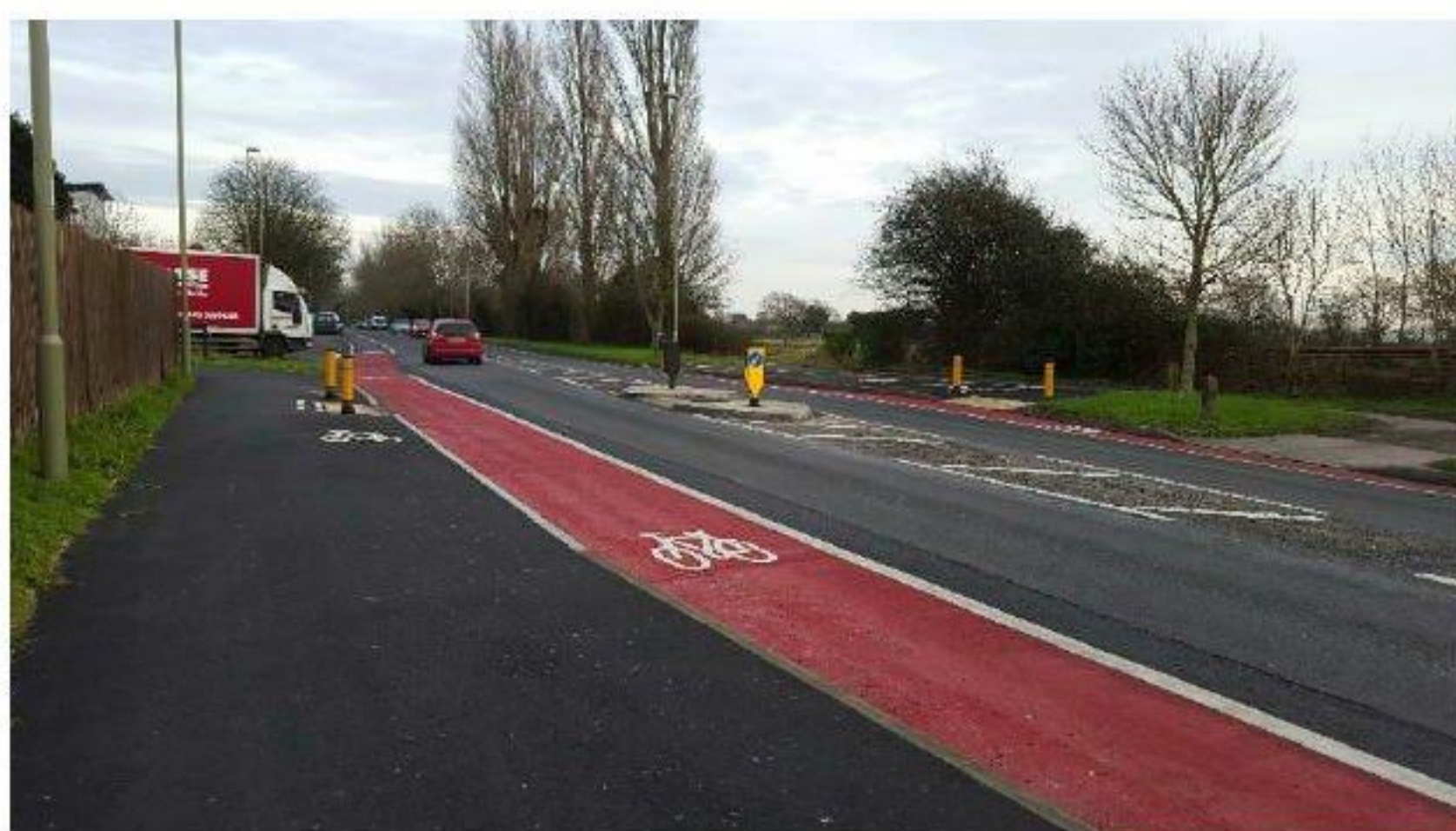
Photograph 5: Recently Upgraded Pedestrian Refuge Island on Havant Road
