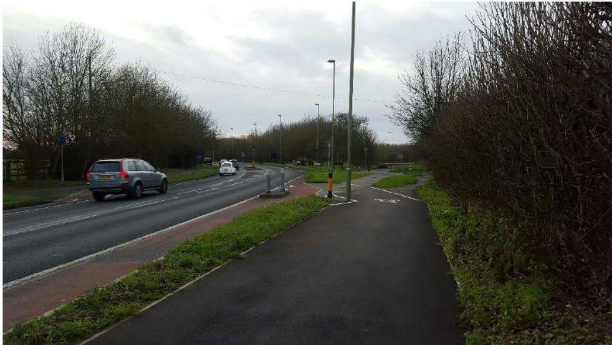
Photograph 6: Recently Upgraded Shared Footway/ Cycleway to the west of the Site
