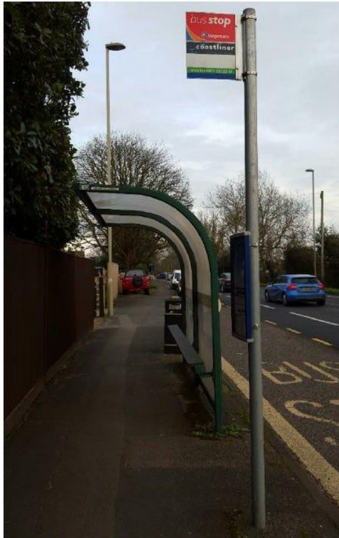
Photograph 8: Havant Road Bus Stop
