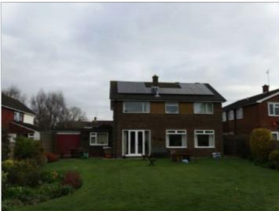
Photo 2 - Rear (South) elevation.
