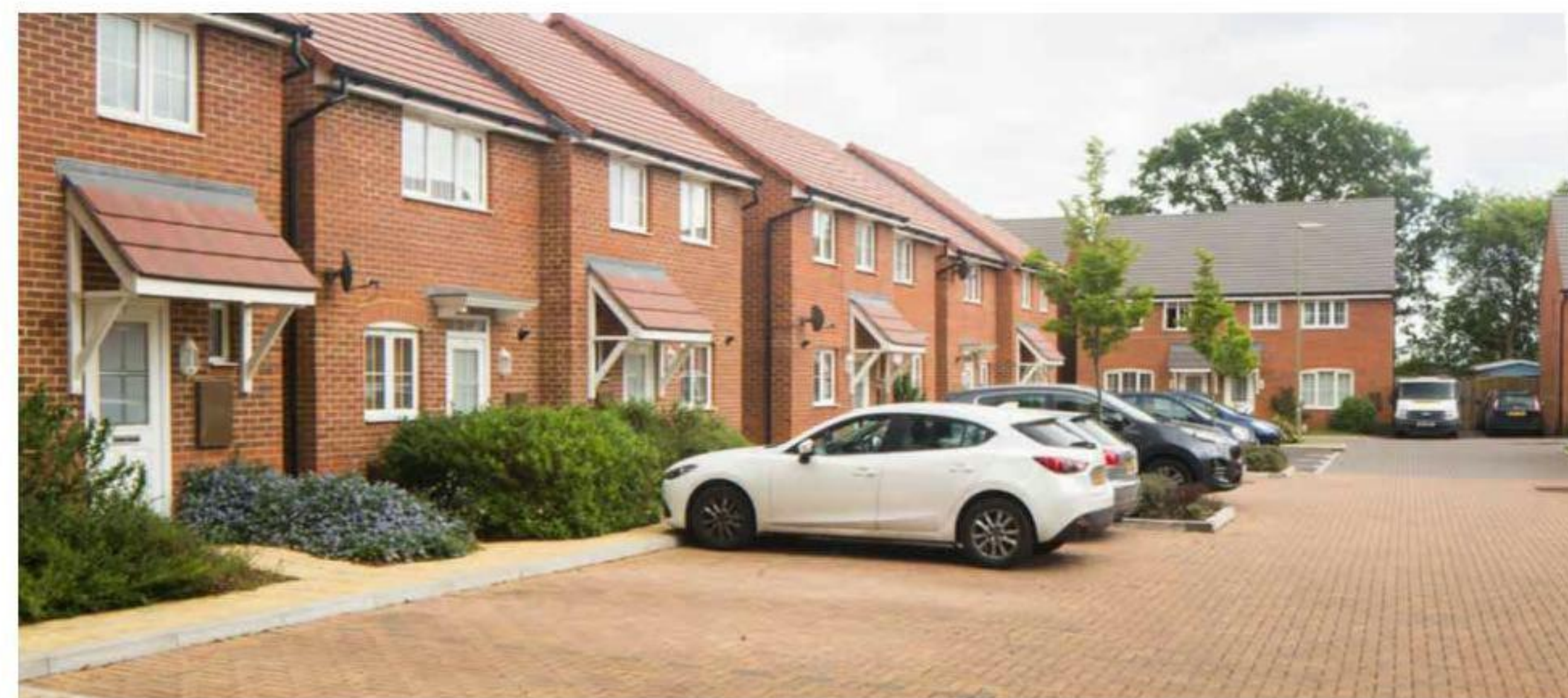
Examples of Permeable Paving Parking Bays
