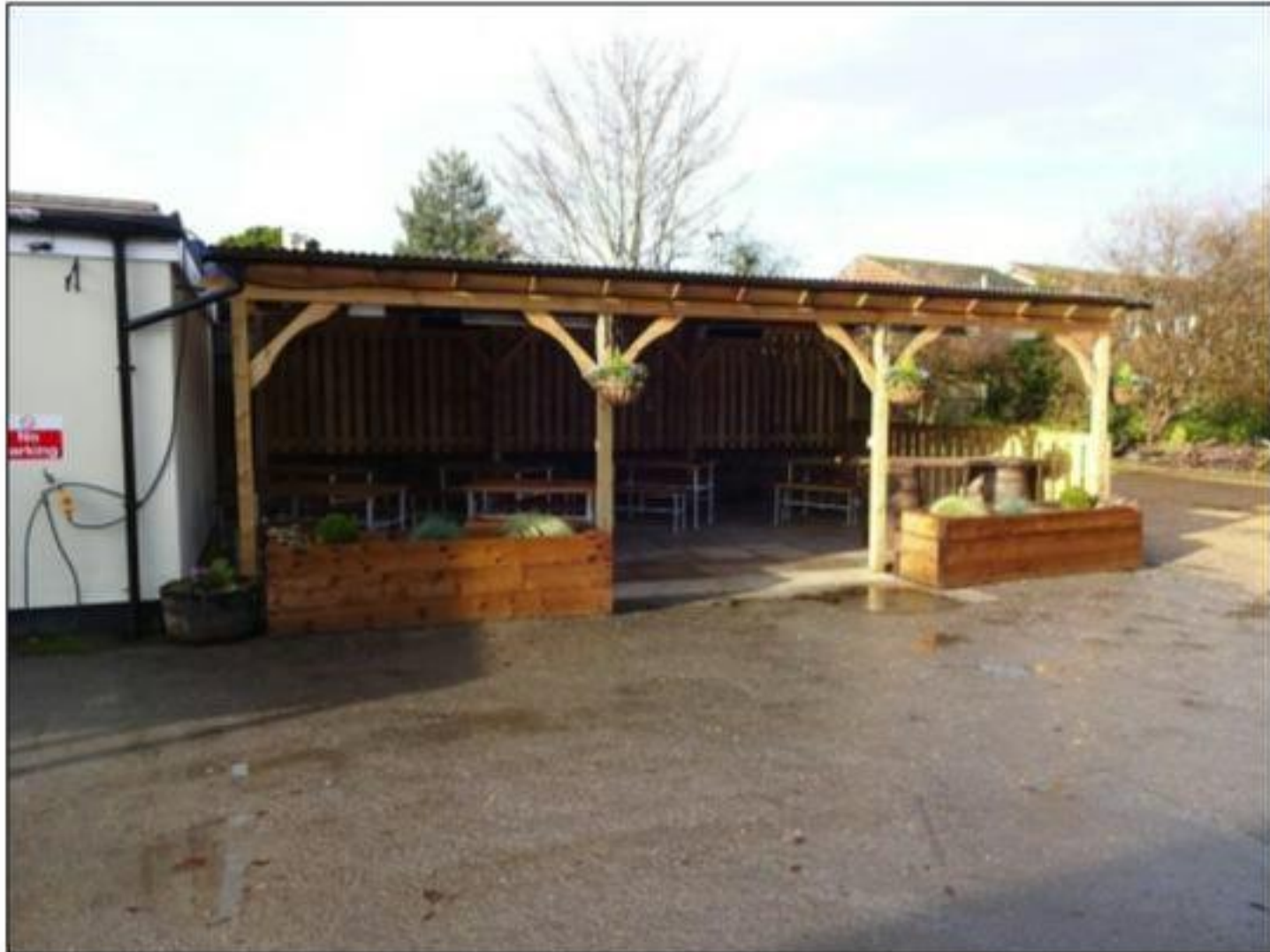
The Kings Arms, new covered seating area
