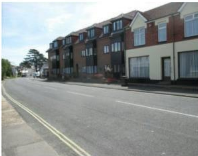
Photograph 4: Station Road Pedestrian Environment
