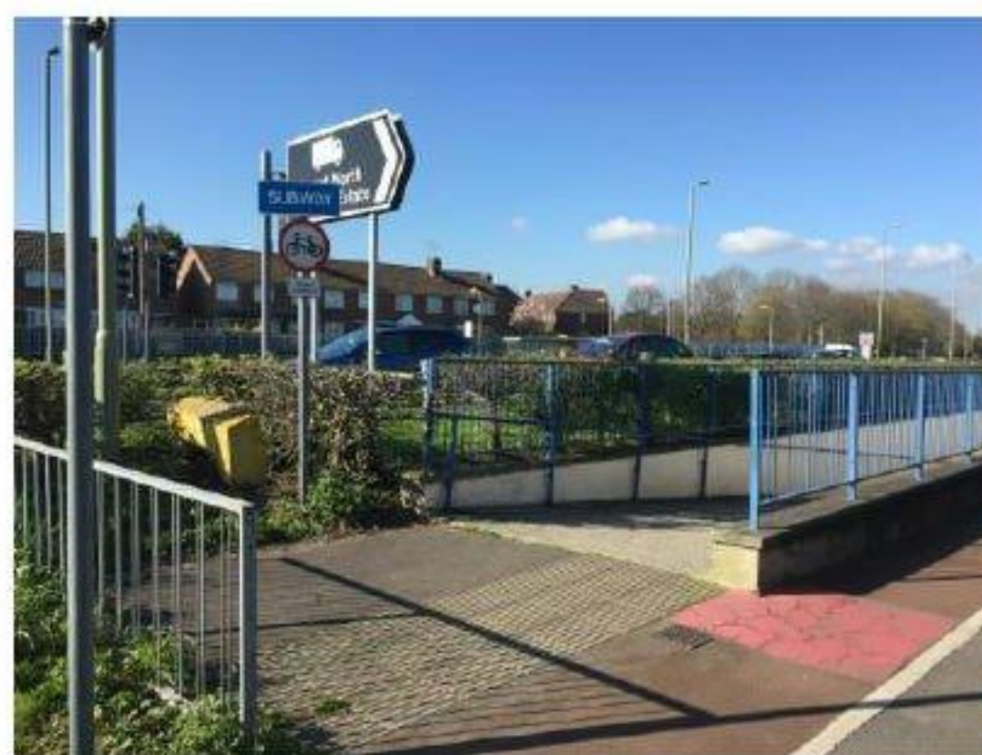
Photograph 5: Underpass on Petersfield Road
