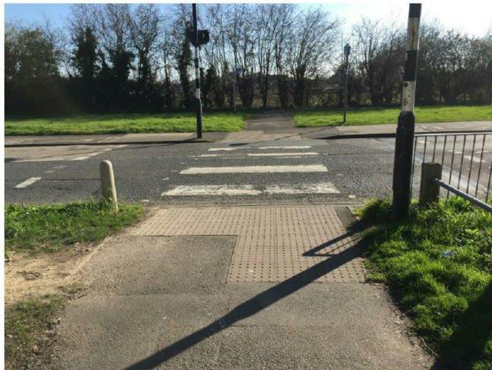
Photograph 3: Pedestrian Crossing on Crossland Drive
