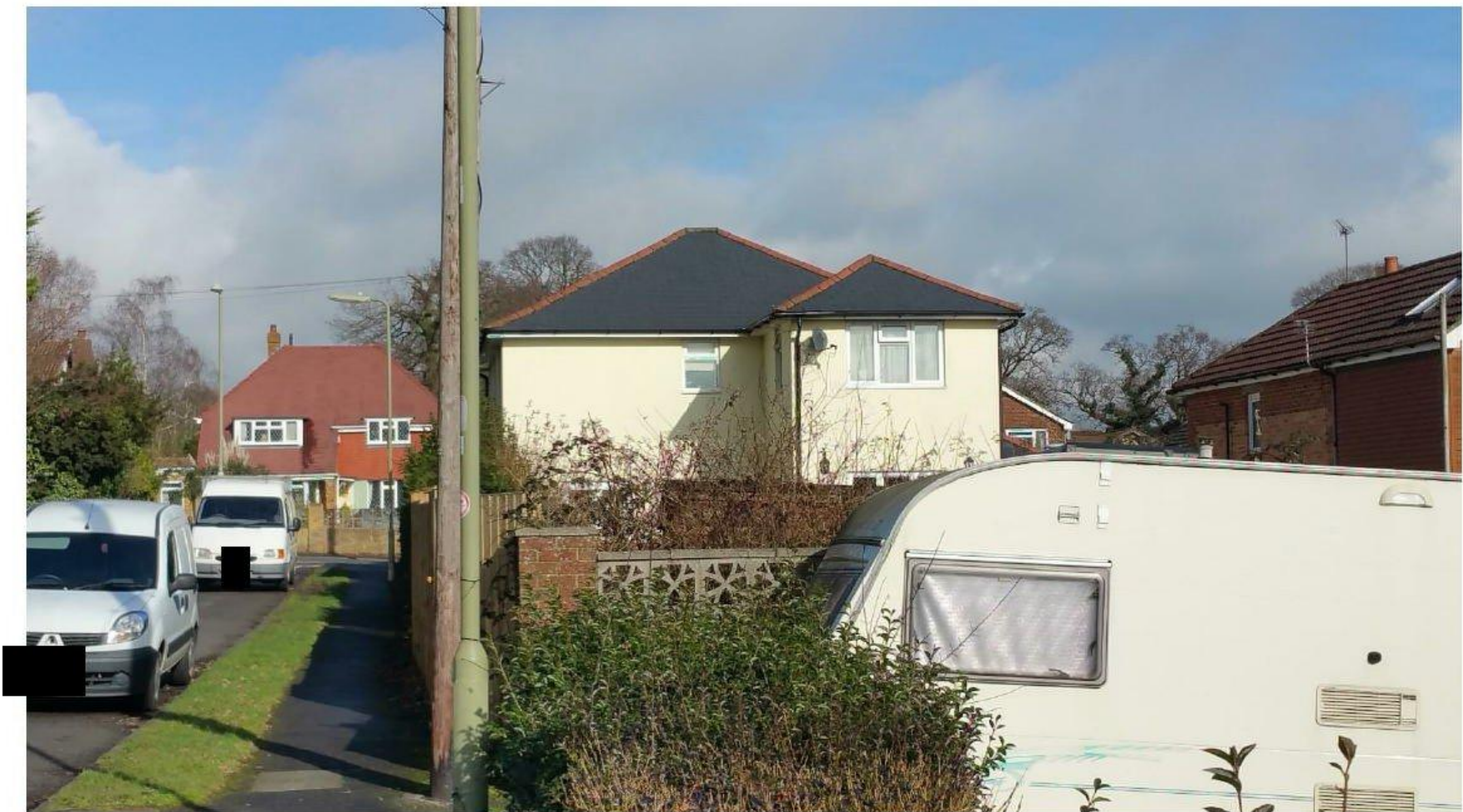
Rear of 17 Lovedean Lane and boundary of 60 Gladys Avenue in the foreground. The proposed property would be squeezed in between the caravan and the rear of No 17 Lovedean Lane
