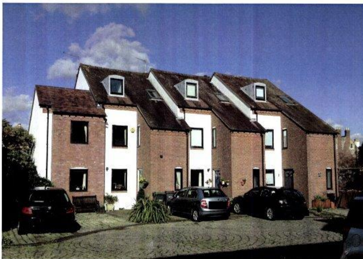
The building group to the North comprising nos 1, 2 and 3.
