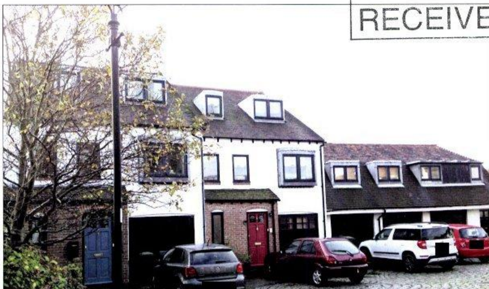
The building group to the South with no 4 to the left, no 5 with the red door in the centre and no. 6 a mews flat above the garage block
